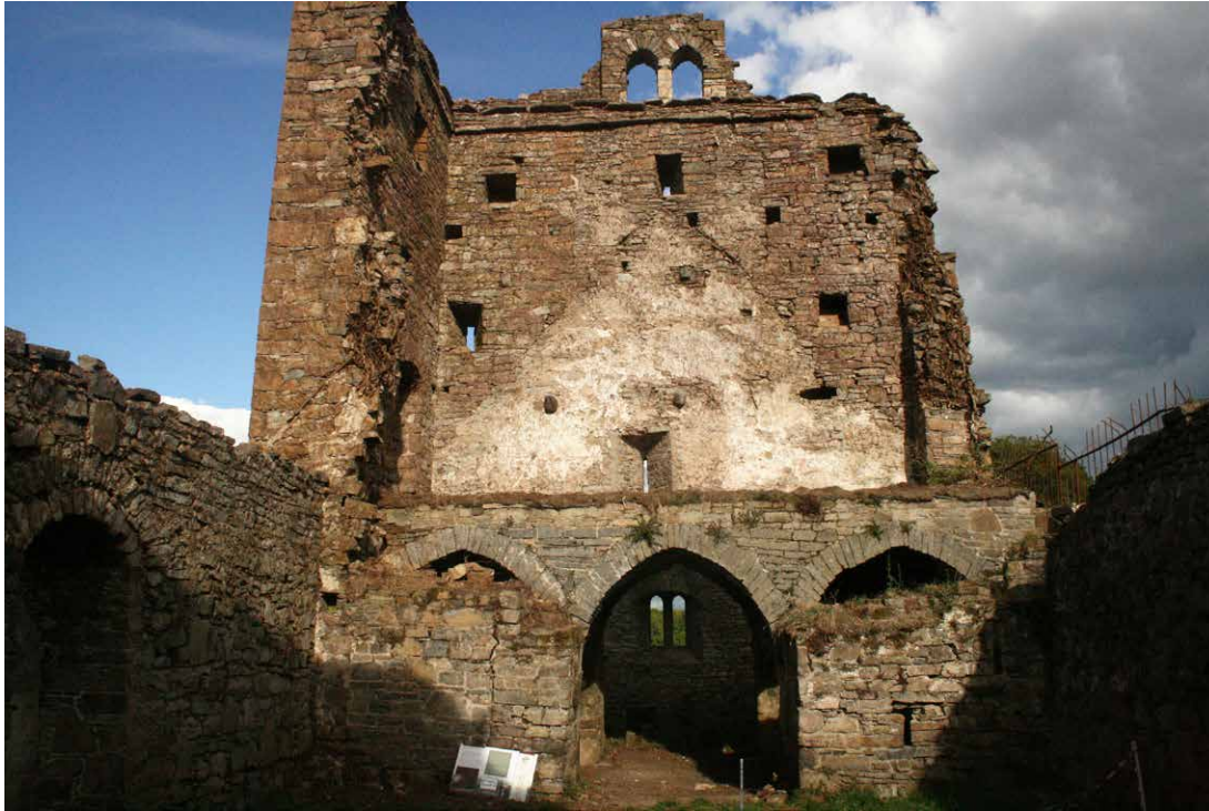
Fig. 5: The pulpitum and residential tower of the parish church viewed from the nave; note the earlier bellcote in the original gable (© Ian Doyle).
