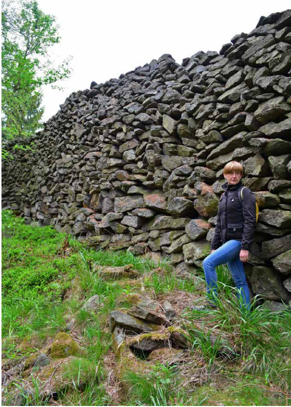
Fig. 2: Kopaniec: an extra-high disposal wall in the southern part of the village (© Paweł Duma).
