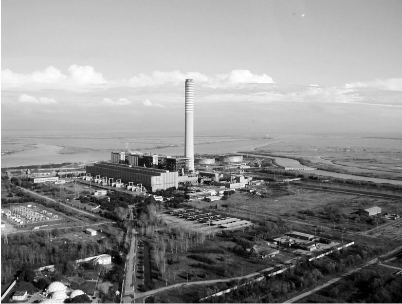
FIGURE 14.3 The power station of Porto Tolle, located in the Po River delta. Source: Enel Produzione S.p.A.
