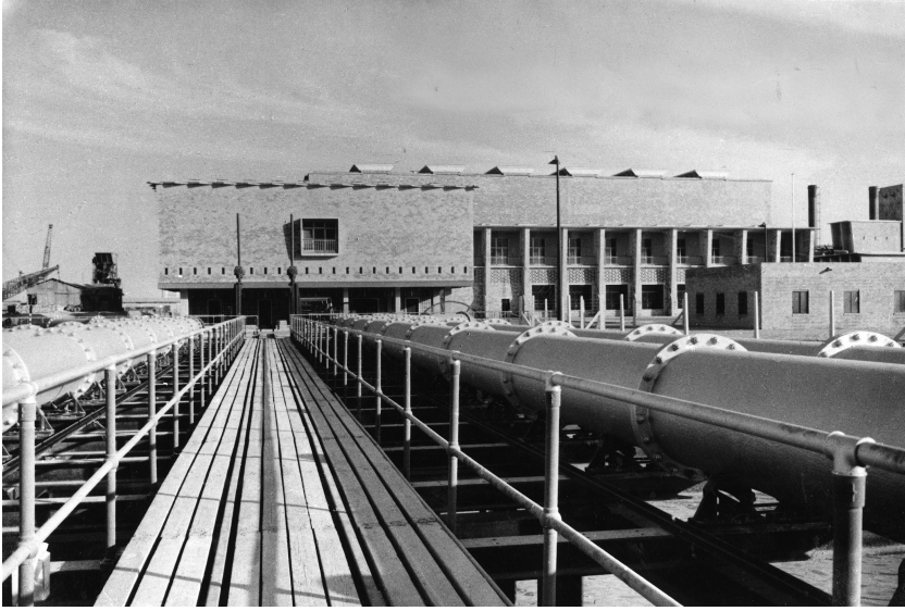
FIGURE 9.2 Administration building with water intake (left) and “Power Station A,” as viewed from the water intake jetty. Source: Unknown photographer, c. 1956, RIBA Collections, RIBA112508.
