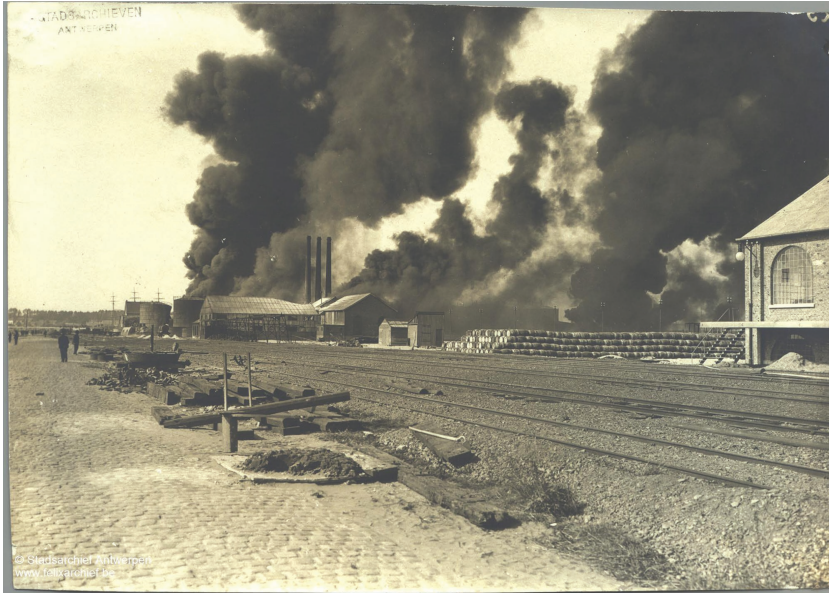
FIGURE 13.7 Petroleum tanks on fire in Petroleum Zuid in 1904. Some of the burning petrol spread toward the Scheldt, but was stopped by the digging of canals. City Archives, Antwerp.
