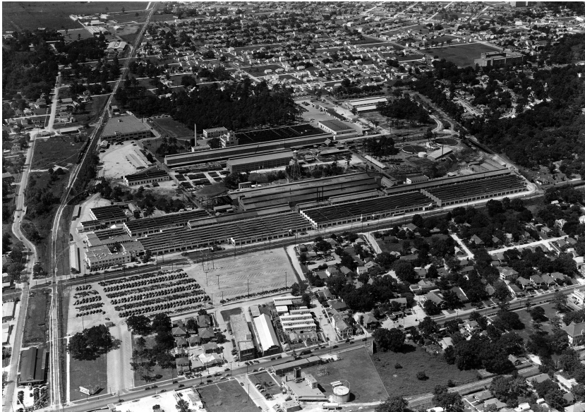
FIGURE 2.10 Aerial photo of Houston's Hughes Tool plant, 1941, a famed example of the numerous oil industry equipment firms located along the Houston Ship Channel. Such firms attracted migrants from small towns and rural areas across Texas and the South. Courtesy of Bob Bailey Studios Photograph Collection, e_bb_3158, Dolph Briscoe Center for American History, University of Texas at Austin.
