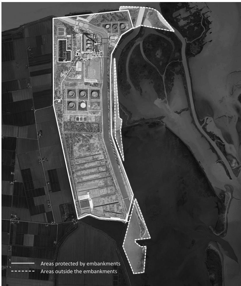
FIGURE 14.7 The power station of Porto Tolle. Source: Google Earth. Image © 2016 TerraMetrics – Data SIO, NOAA, US Navy, NGA, GEBCO modified by the authors.
