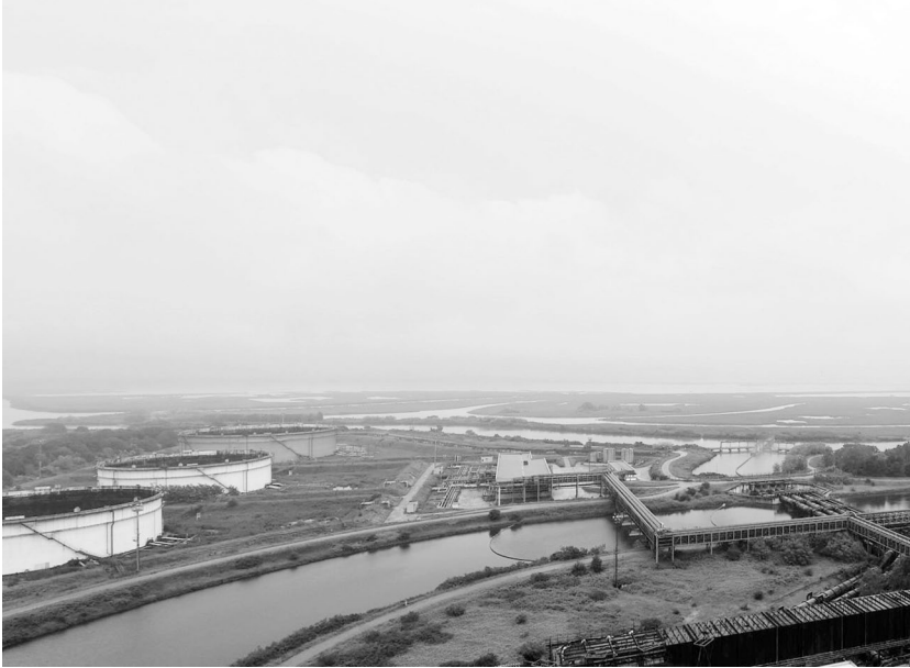
FIGURE 14.15 Oil tanks and view of the two canals used for plant cooling. Source: Chiara Geroldi.
