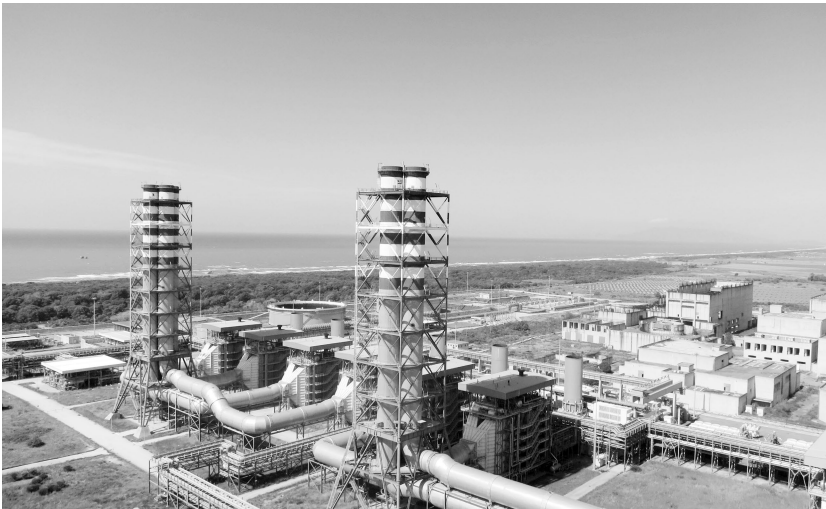
FIGURE 14.4 The power station of Montalto di Castro, located in a former Etruscan territory on the Tyrrhenian Sea. Source: Enel Produzione S.p.A.
