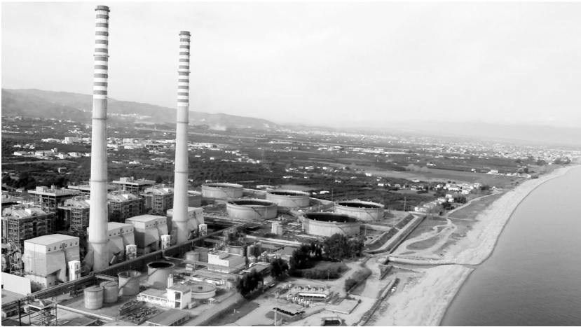
FIGURE 14.5 The power station of Rossano, located on the Ionian Sea. Source: Enel Produzione S.p.A.
