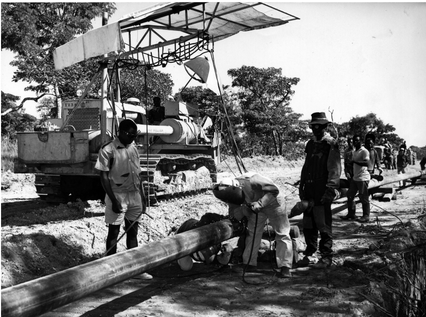
FIGURE 5.12 Construction of the TAZAMA pipeline, Tanzania 1966. Source: ENI Historical Archive.
