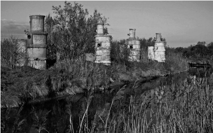
FIGURE 14.9 Abandoned methane gas extraction wells in Ca' Pisani (Porto Viro, RO). Source: Moreno Bonifacio.
