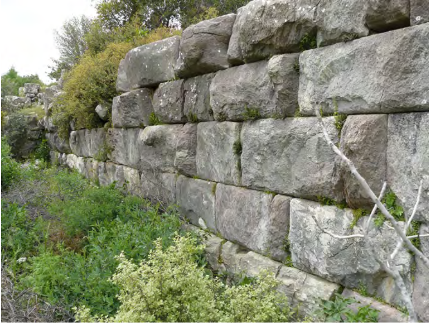
FIGURE 4.9 Southeast corner of the sanctuary with the fourth century temenos wall, showing the ashlar construction with headers and stretchers
