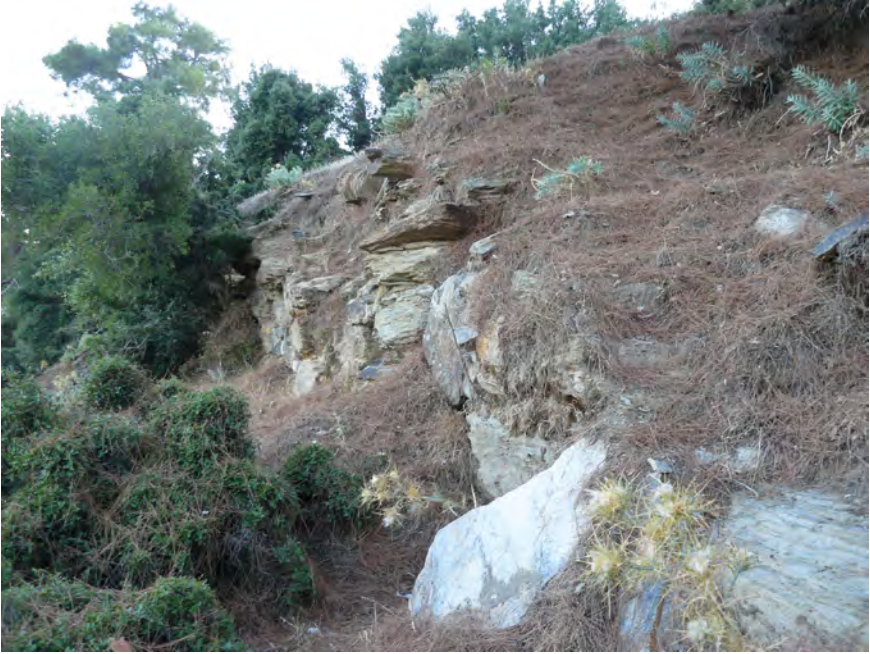
FIGURE 6.13 Panamara. Rock and schist wall along the northeastern perimeter PHOTO AUTHOR 2010
