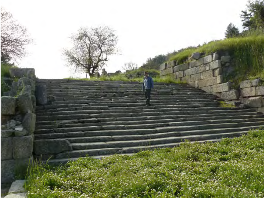
FIGURE 3.7 Labraunda. Monumental staircase leading to the Middle Terrace PHOTO AUTHOR 2008
