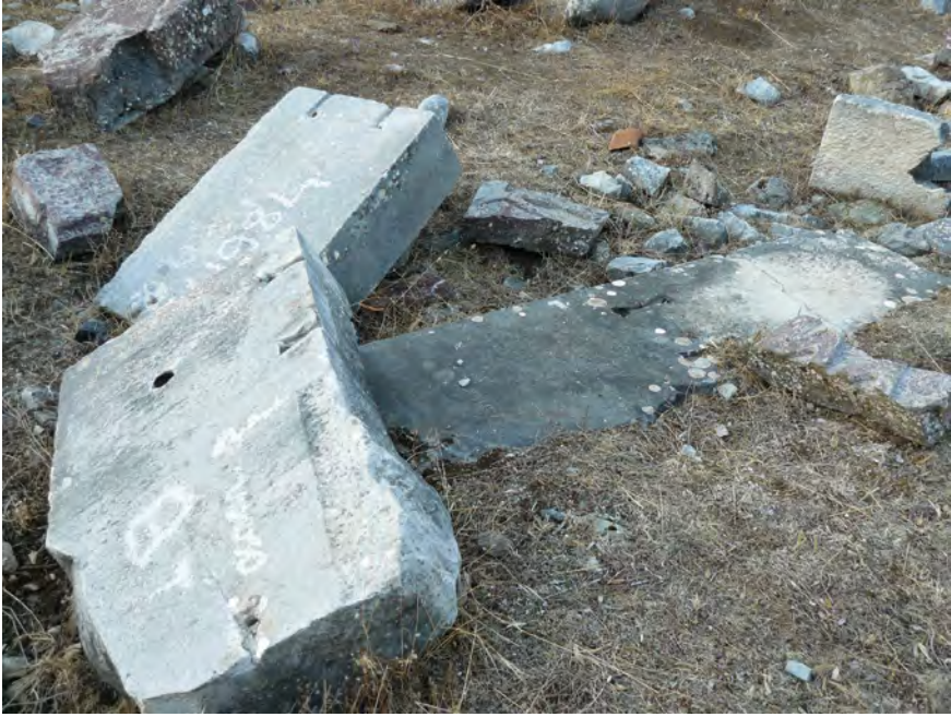
FIGURE 4.14 Sinuri. The eastern stoa. Section of the stylobate, with holes for dovetail clamps
