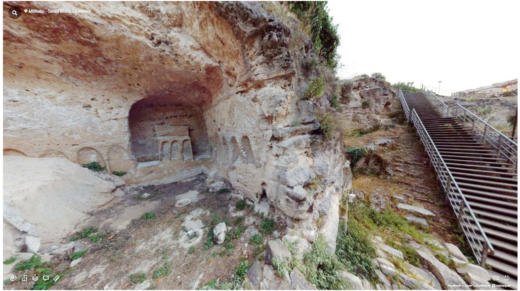
Fig. 8. The pre-existing rock oratory, image taken from the Matterport model. Elaboration by the author.
