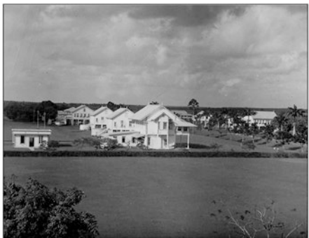
B. The British overseer's quarters at Blairmont Sugar Estate, British Guiana
