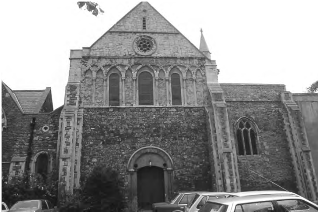
Fig. 7 The west front of St James's Church showing the Norman circular window and arcading. Church House is on the far left of the photograph.
