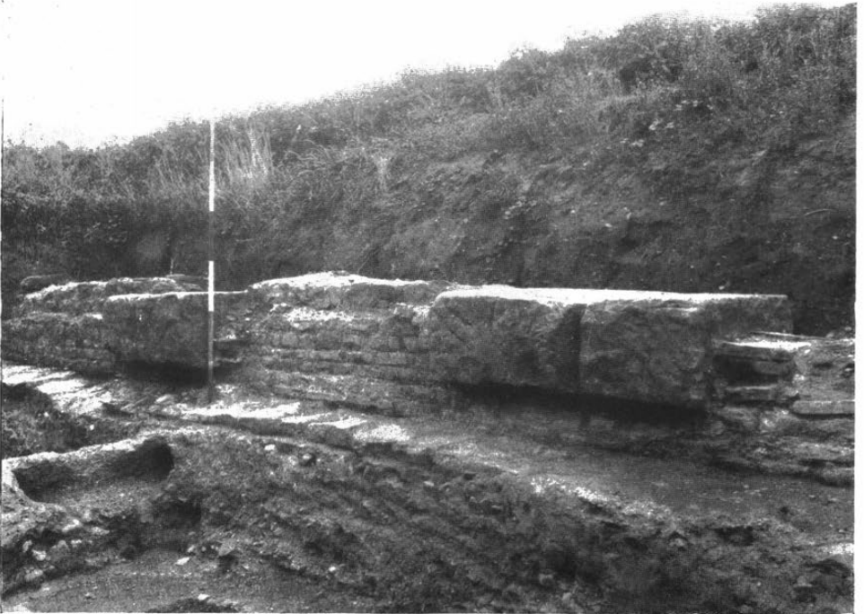
Fig. 2. Foundations of portico, site VI. p. 8
