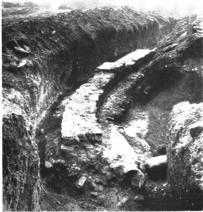
Fig. 1. Foundations of outer wall, north-east corner of site VII. p. 20
