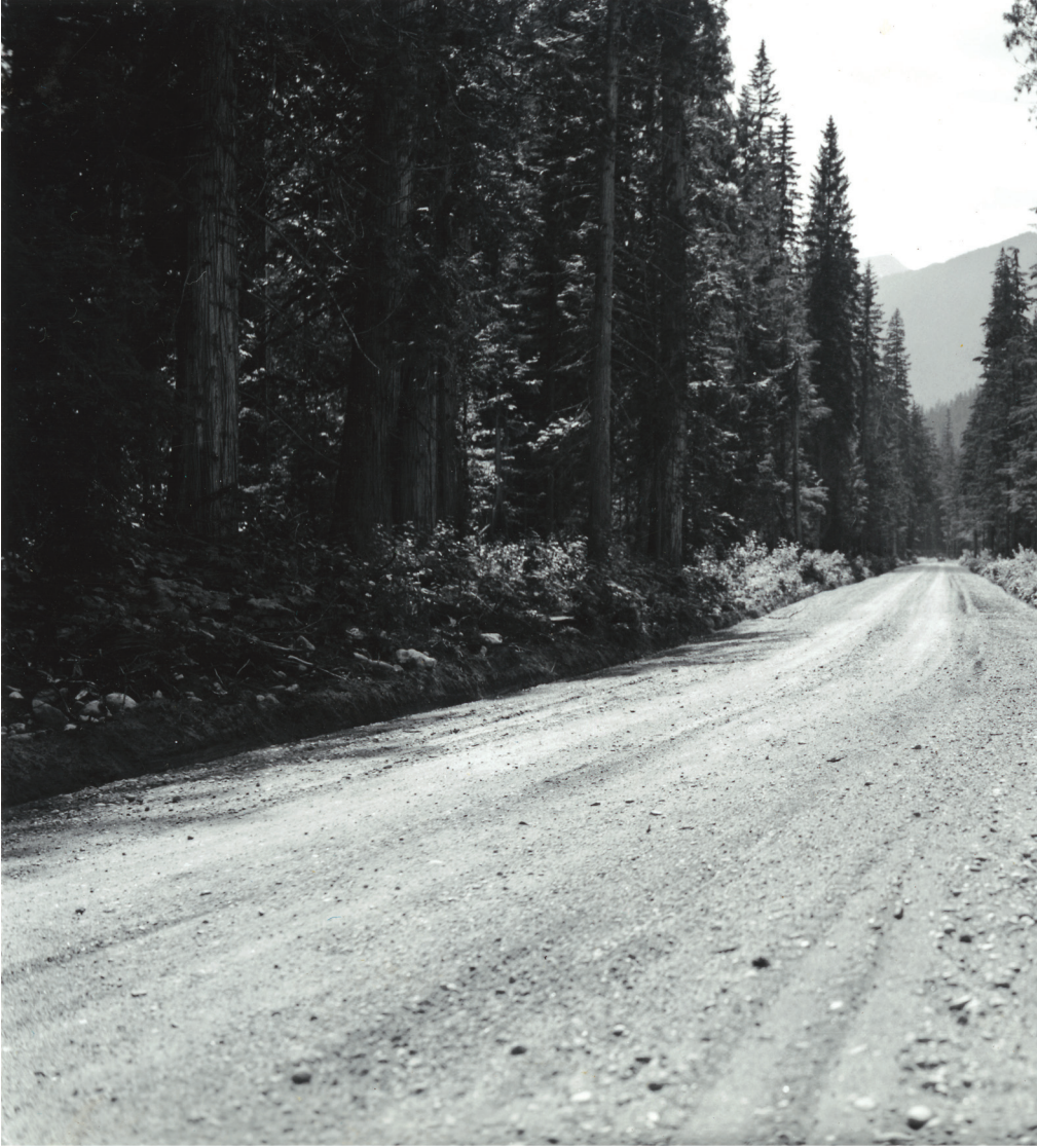
FIG. 3. GOLDEN REVELSTOKE HIGHWAY, BASE STA 240 + 100 LOOKING WEST, BIG BEND HIGHWAY, AUGUST 1939. [SOURCE: LIBRARY AND ARCHIVES CANADA, PARKS CANADA COLLECTION/EO10836789.]
