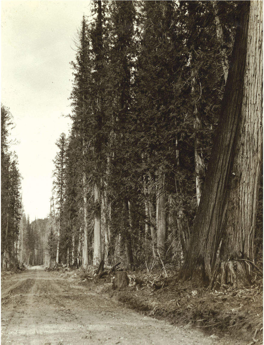
FIG. 2. NEW GRADE AND BIG TIMBER AT BOULDER CREEK, BIG BEND HIGHWAY. [SOURCE: LIBRARY AND ARCHIVES CANADA, PARKS CANADA COLLECTION/e010836790.]
