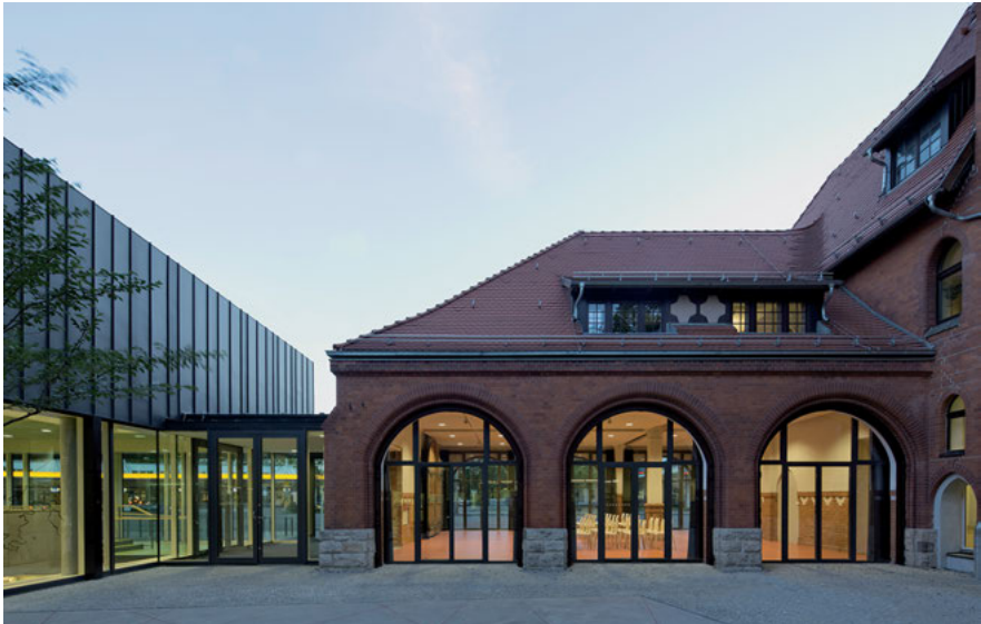
Fig. 5: The library courtyard and old fire engine hall. © Werner Huthmacher.
