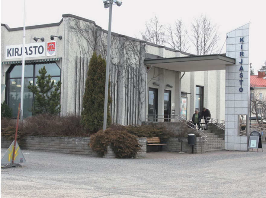
Fig. 1: The Joutsa Public Library moved into a renovated former grocery store from the late 1970s. © Eero Peltoniemi.
