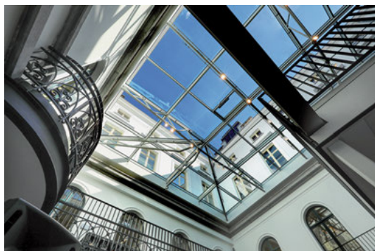
Fig. 7: One of the inner courtyards creating an atrium. © Hilde Christiaens.
