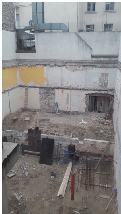
Fig. 2: Demolition of the old courtyard. © AUP.
