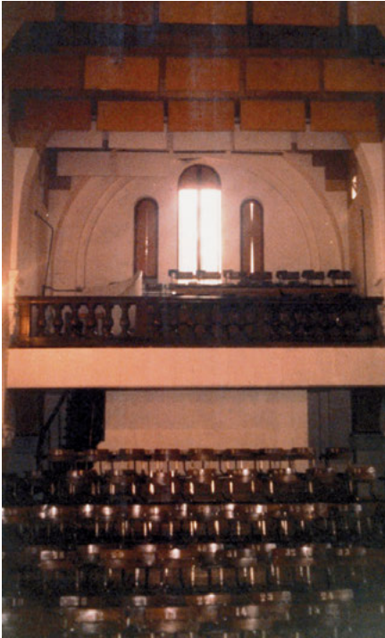
Fig. 3: View before the refurbishment. © Antonio Castañeda Buraglia.
