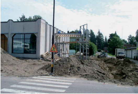
Fig. 4: The biggest external structural change: the main entrance relocated to a safer location in the side street. © Eero Peltoniemi.
