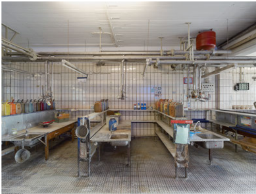
Fig. 13: The abandoned original dyeing room. © Wolfram Janzer.
