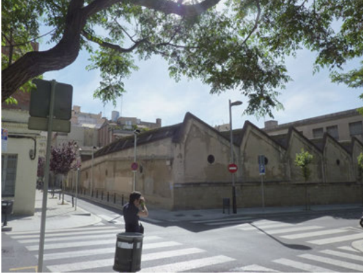
Fig. 8: Initial building. © Ricard Mercadé Aurora Fernández arquitectes.
