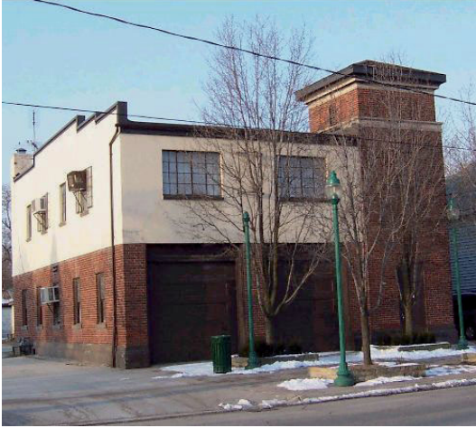
Fig. 3: View of Fire Hall No. 6 before renovations. © City of Windsor, Nancy Morand.
