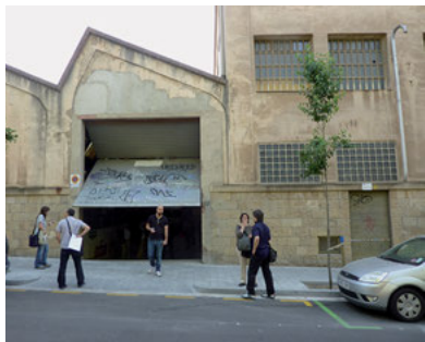
Fig. 12: Original building. © Ricard Mercadé Aurora Fernández arquitectes.
