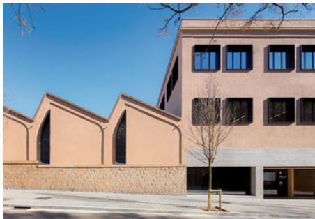
Fig. 13: Completed project. © David Cardelús.
