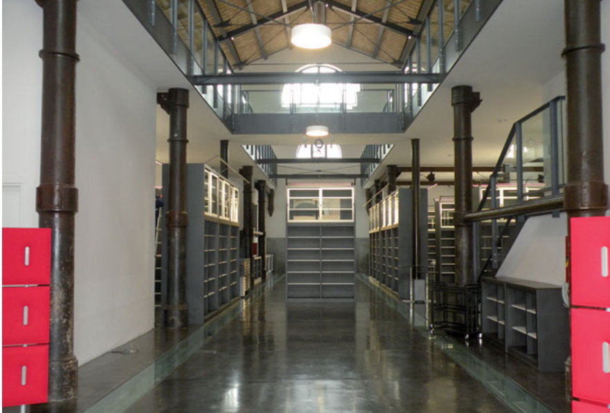
Fig. 9: Internal of the Pavilion 9E after restoration: the roof rebuilt and the iron elements as structures of the new mezzanine. © Anna Raimondi.
