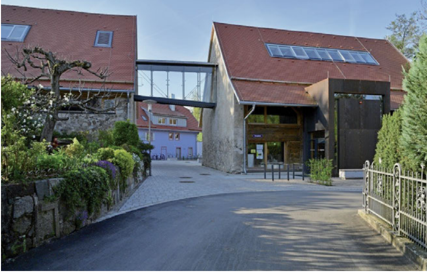
Fig. 1: The transformed Talvogtei barns viewed from the north with the Multimedia Centre on the right and administration centre and community hall on the left. © Willi Loba.
