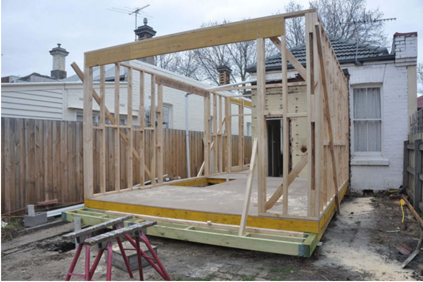
Figure 28. Avery Green during construction. Photograph by Pia Ednie-Brown, 2015.
