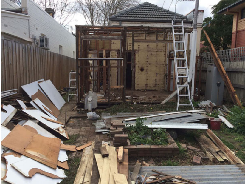
Figure 27. Avery Green during Demolition phase. Photograph by Pia Ednie-Brown, 2015.
