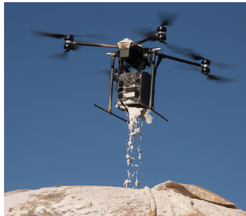
2. Drone depositing a coat over a large inflatable dome. Barcelona Drone Center, 2018. Photo: Frederic Carmona.
