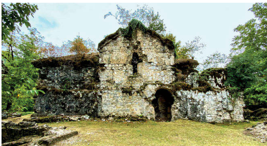
Fig. 18: Yeddi Kilsə. Eastern church. North façade.
