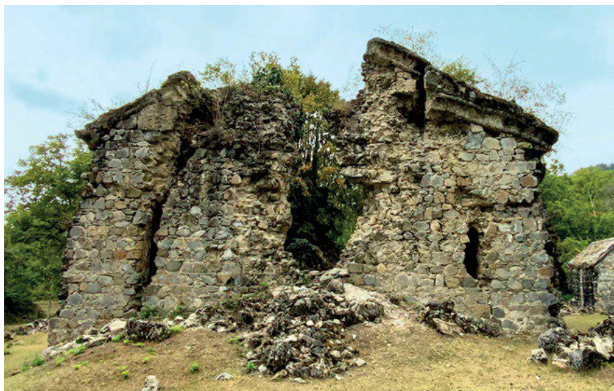
Fig. 19: Yeddi Kilsə. Eastern church. East façade.
