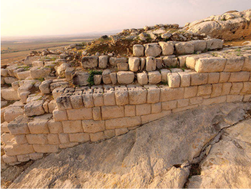
Fig. 7: Horizontal polished surfaces of the quadras, rustic elaboration of the outer faces, facets and “swallow-tail” connections of the northern fortification wall, 2009.
