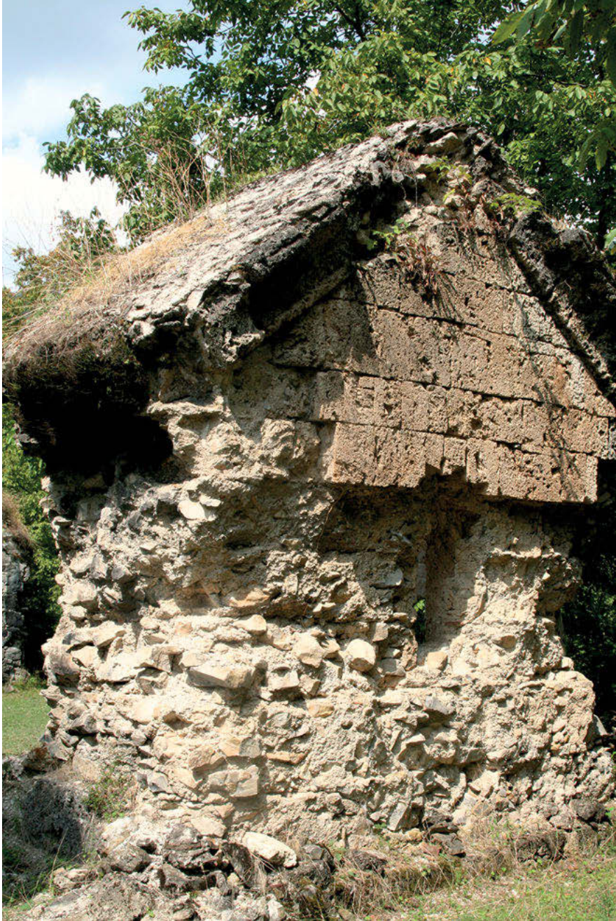
Fig. 26: Yeddi Kilsə. Vestiges of a chapel to the northeast of the eastern church: Eastern façade.
