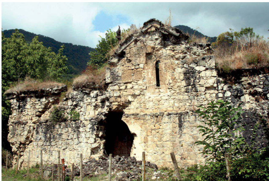
Fig. 17: Yeddi Kilsə. Eastern church. South façade.
