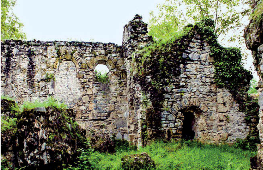
Fig. 8: Yeddi Kilsə. Western church. North wall and northeast sacristy seen from the south.
