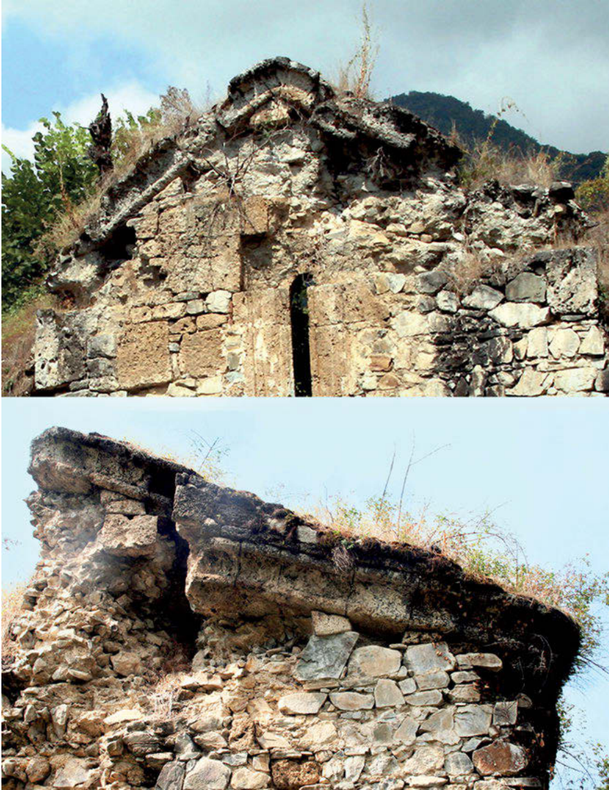
Fig. 20: Yeddi Kilsə. Eastern church. Parts of cornices on south and north gables.
