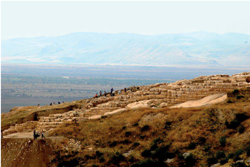
Fig. 5: Upper part of the northern fortification walls, 2009.
