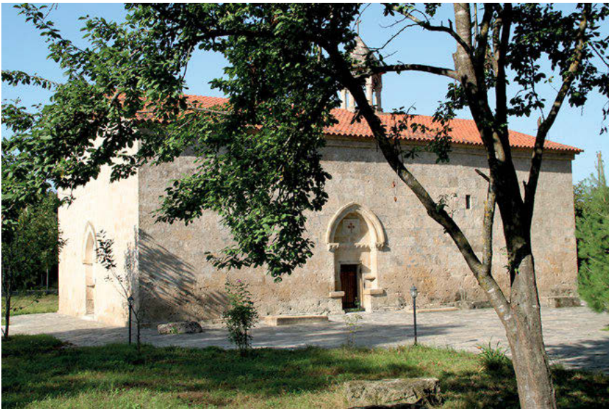
Fig. 3: The Chotari church after its reconstruction (August 2011).
