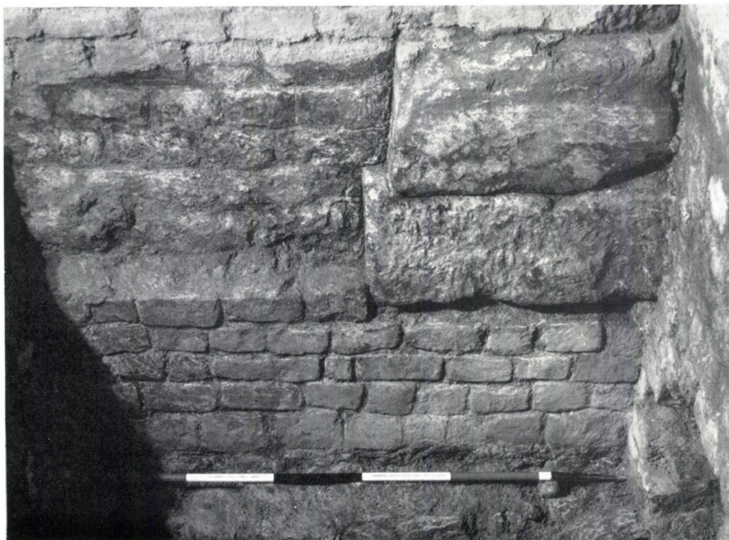
b. Trench 1, south of the Circular Bath, showing the north wall of the first-period bath with the second-period wall on top (p. 135)
