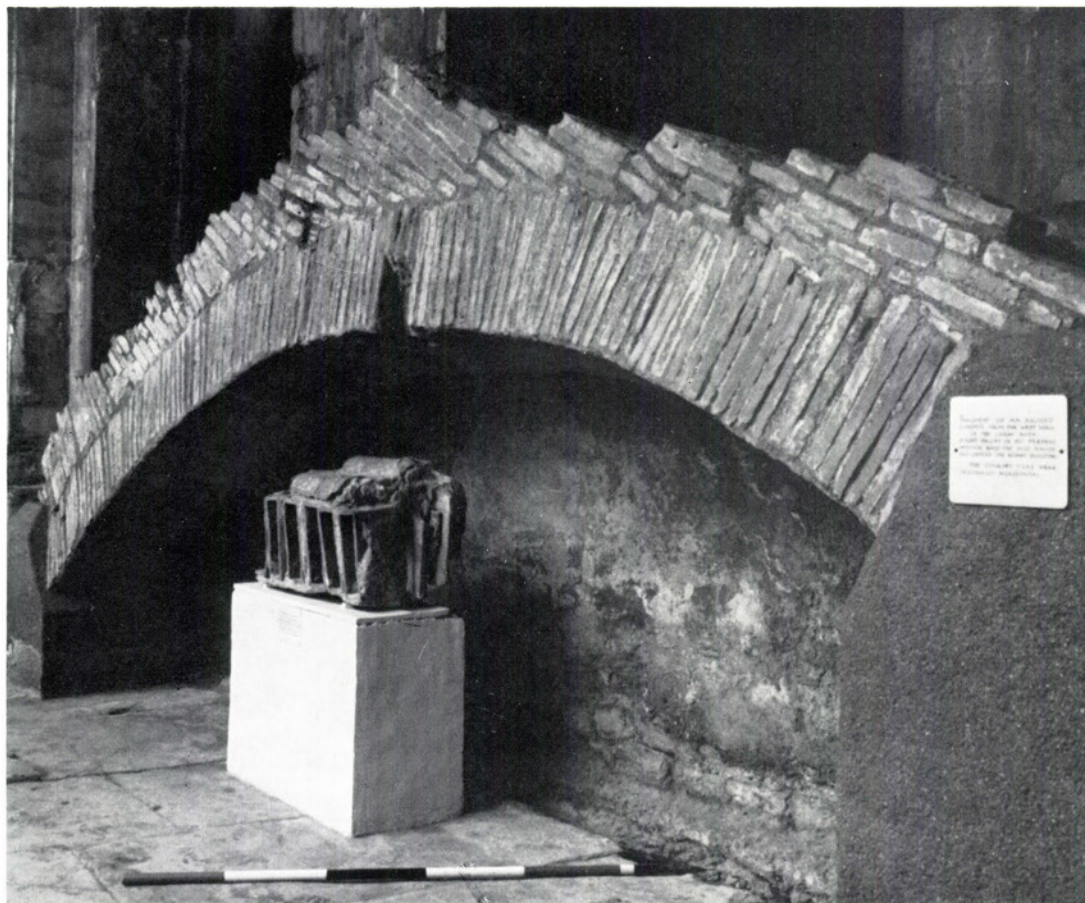
b. The facing of the vaulting which once covered the Great Bath (p. 98)
