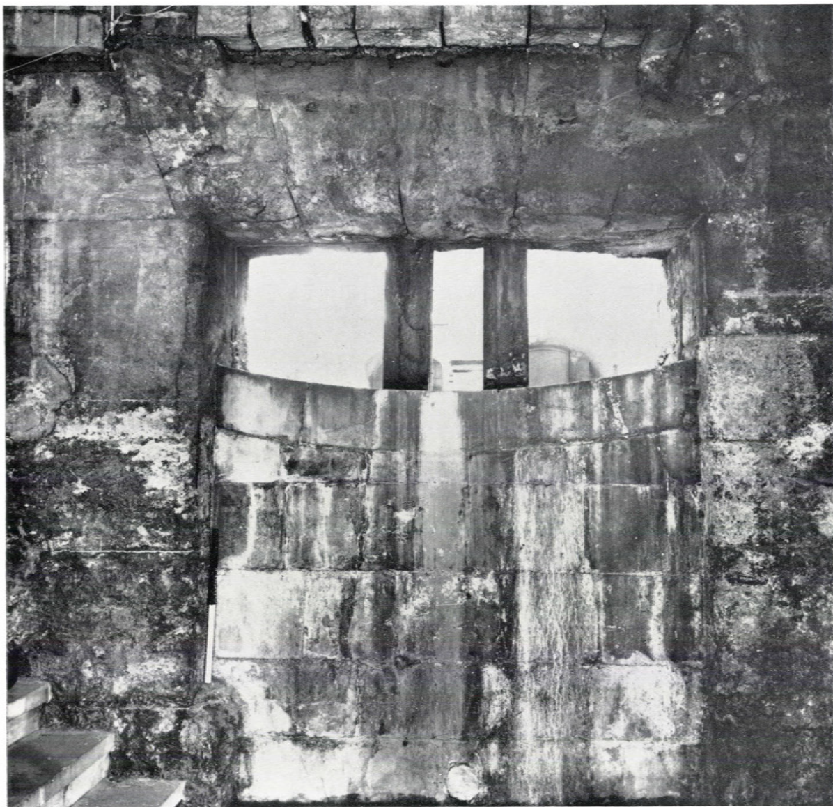
a. Square window opening of first-period date in the north wall of the hall overlooking the Reservoir (cf. fig. 35) (p. 103)
