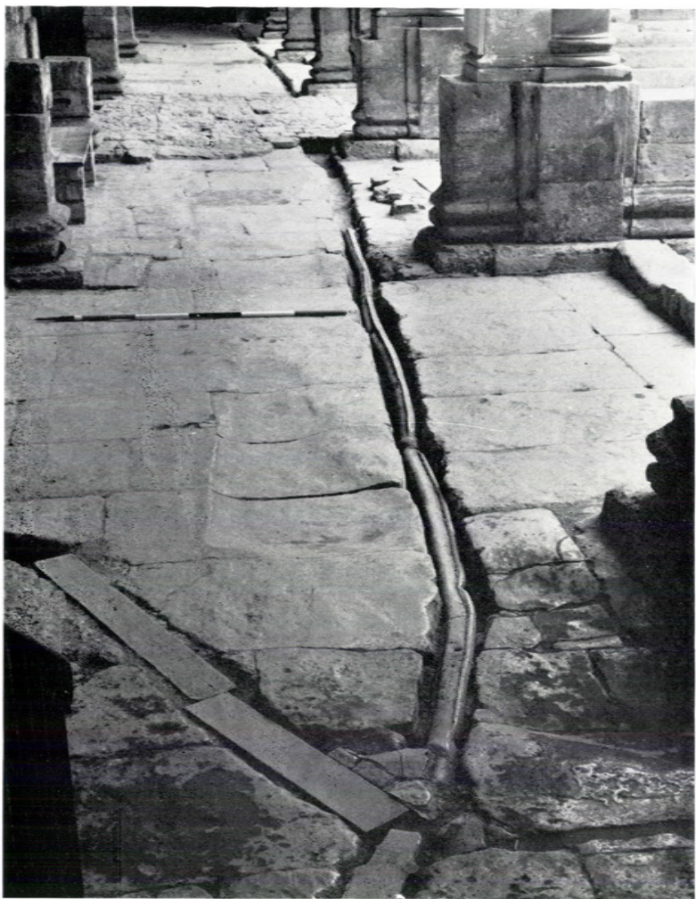
a. The lead pipe in position in the ambulatory of the Great Bath (p. 100)
