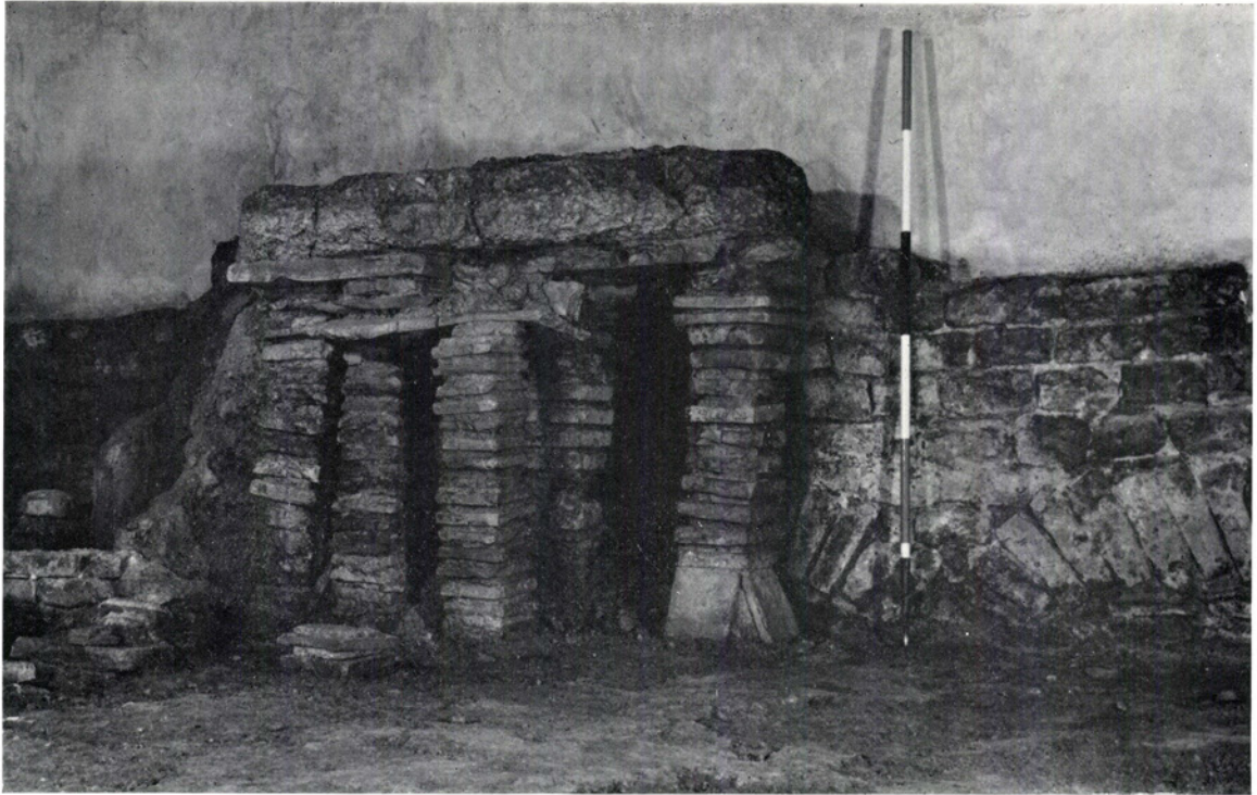
a. The East Baths showing the fourth-period hypocaust. The relieving arches can be seen in the east wall behind (p. 114)
