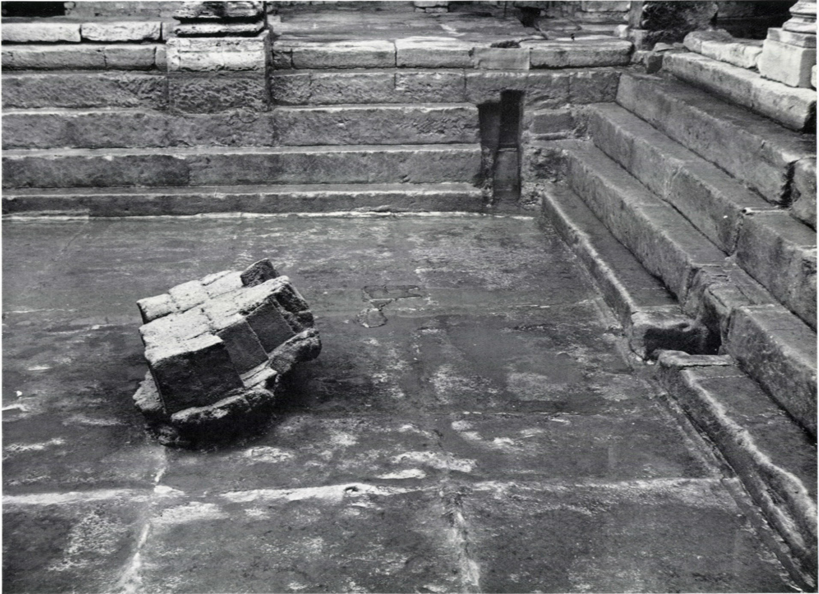
The east end of the Great Bath looking north. The drain sluice can be seen in the north-east corner of the bath. In the centre of the east side is the outfall leading to the Lucas Bath. The mass of masonry lying on the lead sheets is part of the vaulted roof (p. 95)
