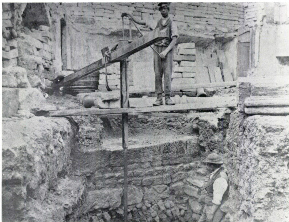
b. The baths beneath the Royal United Hospital showing the excavation in progress, c. 1867 (p. 151). Photograph: Irvine Collection
