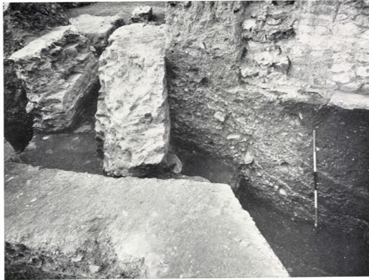
a. Subsidence adjoining drain in south-east angle (p. 21)
