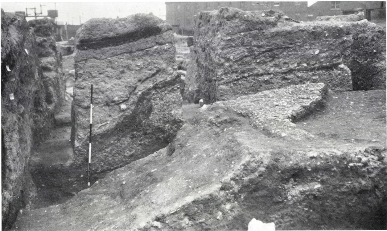
b. Edge of subsidence on south side of Forum from the south (p. 22)
