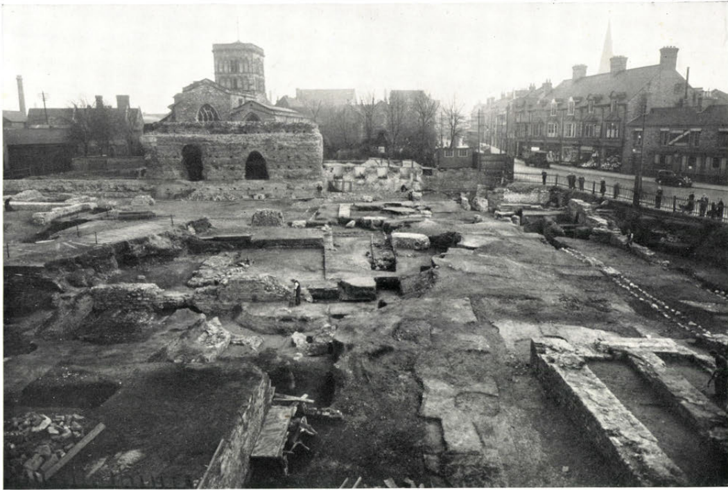
a. General view of the south half of the site from the west
