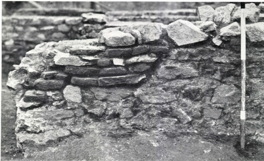
a. Rebuild of south wall of Period IV (water-tank?) building
