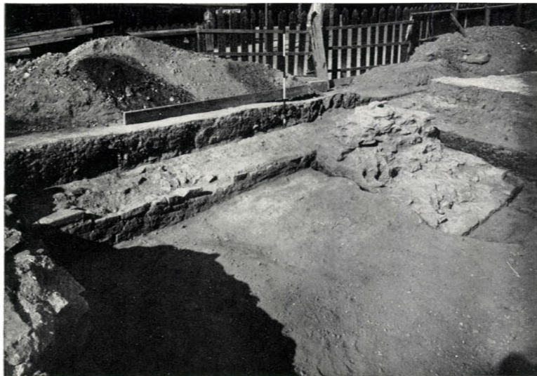
a. North wall of Basilica and north pier of western aisle (p. 14)
