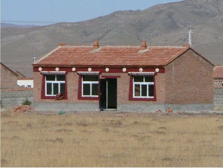
FIGURE 3.3. Nomadic Settlement built by the government in Ningxiu, Zeku County, October 2009
