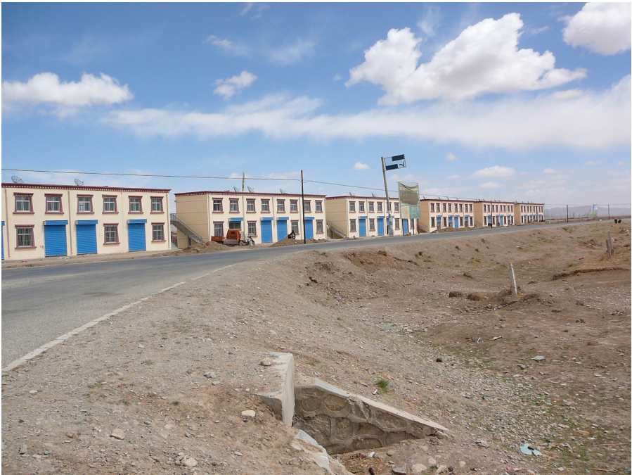
FIGURE 4.4. Ecological Resettlement of rMar stod pastoralists providing two-story apartment complexes, with commercial units on the ground floor and living quarter at the upper level, Tongde County, May 2007
