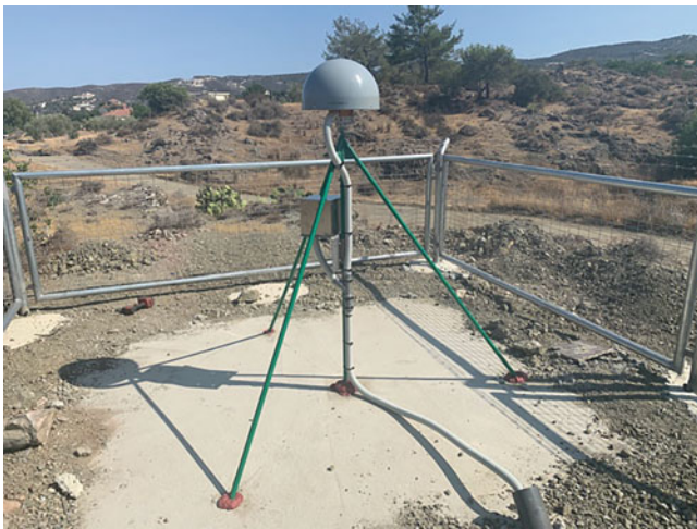
Fig. 3 The shallow drilled braced monument type used in the CyCLOPS PS
