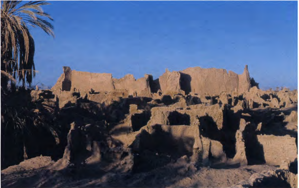
Fig. 1.7. The Jarma kasba (GER 1.65) served only as a date store by the 19 th century.
