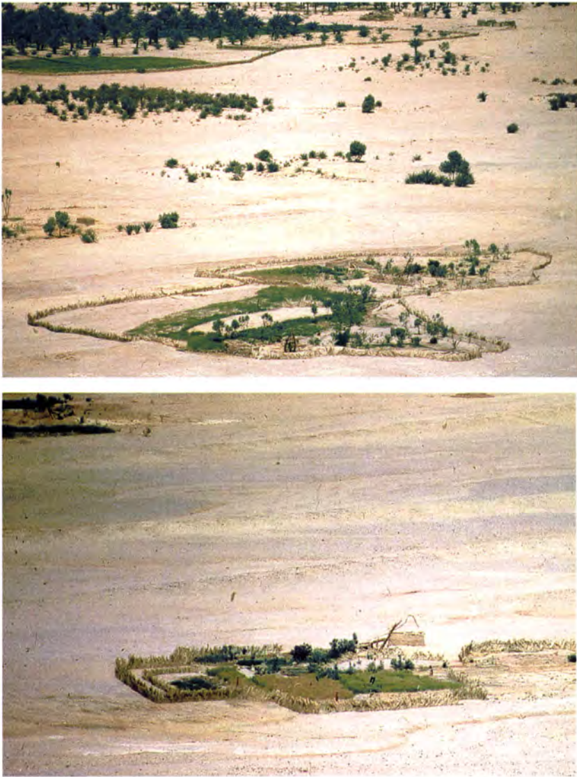
Fig. 9.28. a) and b) Traditional dalw wells (note the A-frame structures) in small gardens (sāniat) that were still in cultivation in the 1960s.
