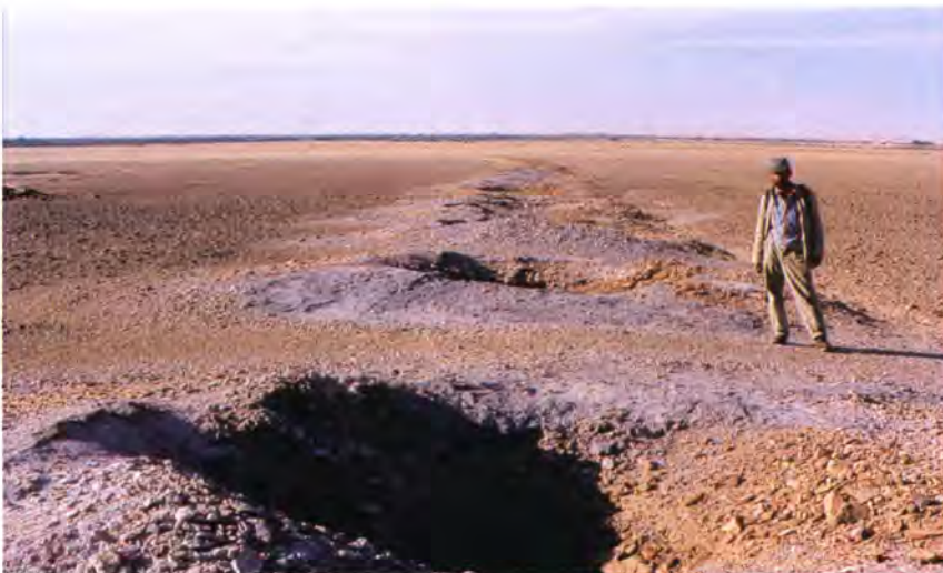
Fig. 7.13. Foggara with closely-spaced access shafts (TAG 8.F207).
