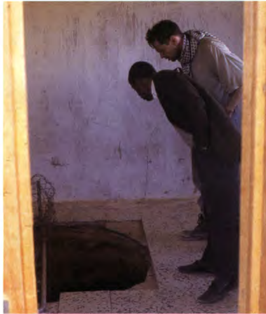
Fig. 7.12. a) Destruction of TWE 16 foggara group by modern bulldozing; b) Qarāqra, floor of bedroom collapsed into foggara shaft.
