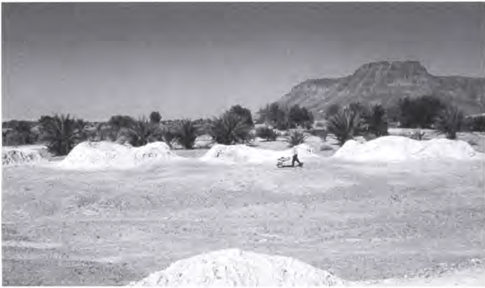
Fig. 7.2. Tuwash foggaras (TWE 16, F13) showing large clay spoil rings.
