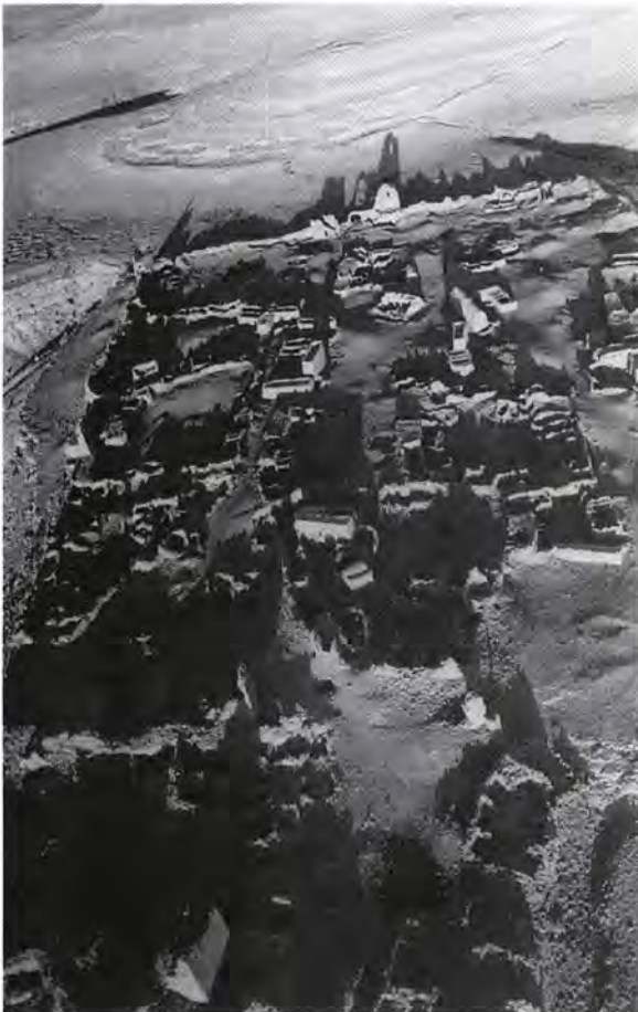
Fig. 3.3. The Roman fort at al-Qurayyāt al-Gharbiya on the central route to Fazzān.
