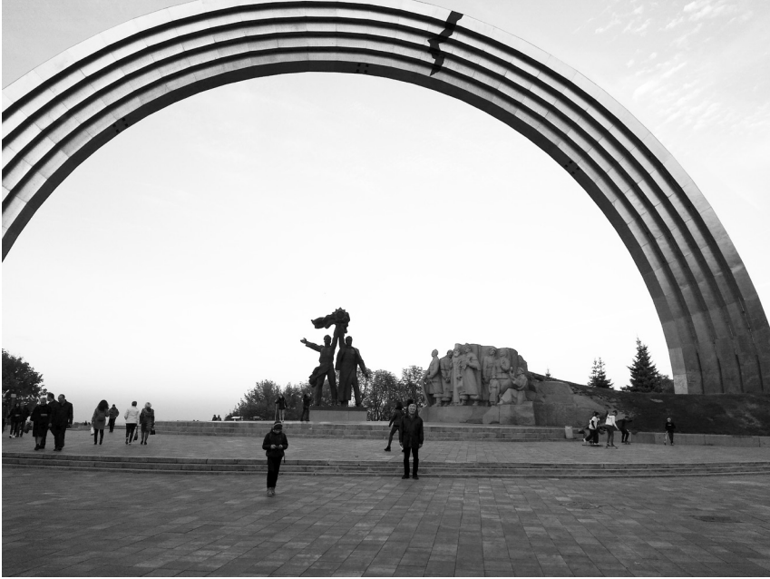
FIGURE C.1. The People's Friendship Arch now includes a crack as symbolic commentary.
