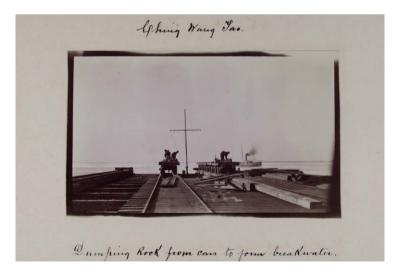
Figure 7 – Ching Wang Tao. Dumping Rock from cars to form breakwater. MS15/6/11E/38.
