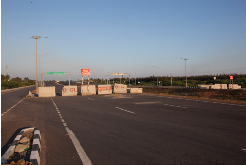
Figure 15.3 Outer Ring Road, Chennai. Source: Christophe Delory.
