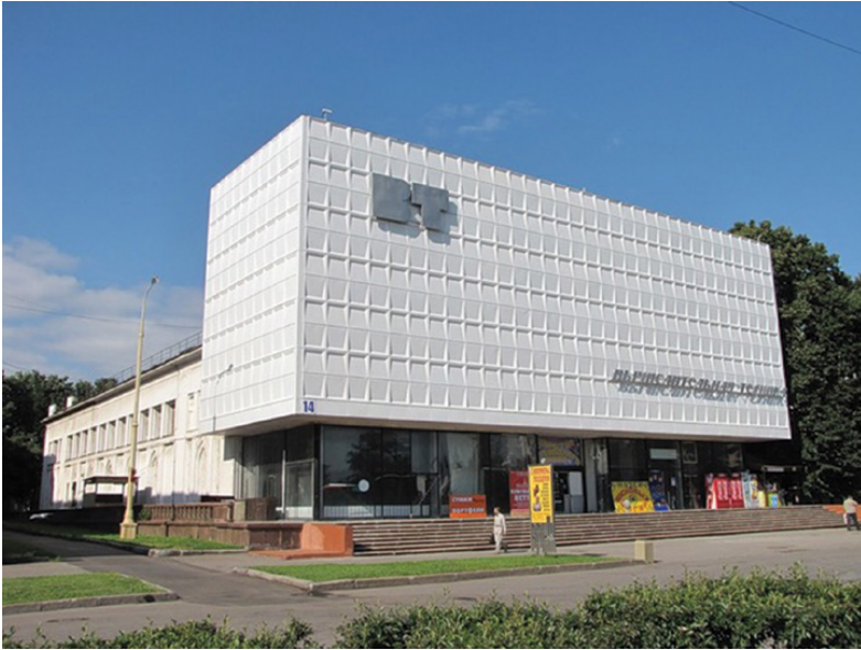
Figure 3.5 Computer Engineering Pavilion between 1967 and 2014. VDNKh. Public domain.
