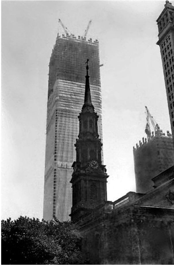
Figure 12.2 Construction of New York's World Trade Center, 1971. Public domain.
