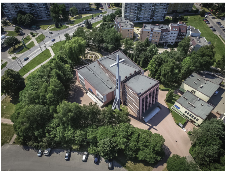
Figure 9.2a and b The Church of St John the Baptist in Tychy (1957–1958) by Zbigniew Weber and Tadeusz Szczesny. The temple appeared before the surrounding structures, preceding the growth of the city. Source: Igor Snopek.
