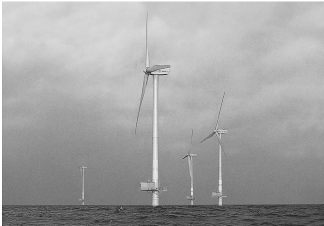
Figure 1.11: Offshore wind farm Utgrunden off the southern Swedish North-Sea coast (7 wind turbines of 1.5 MW each).
