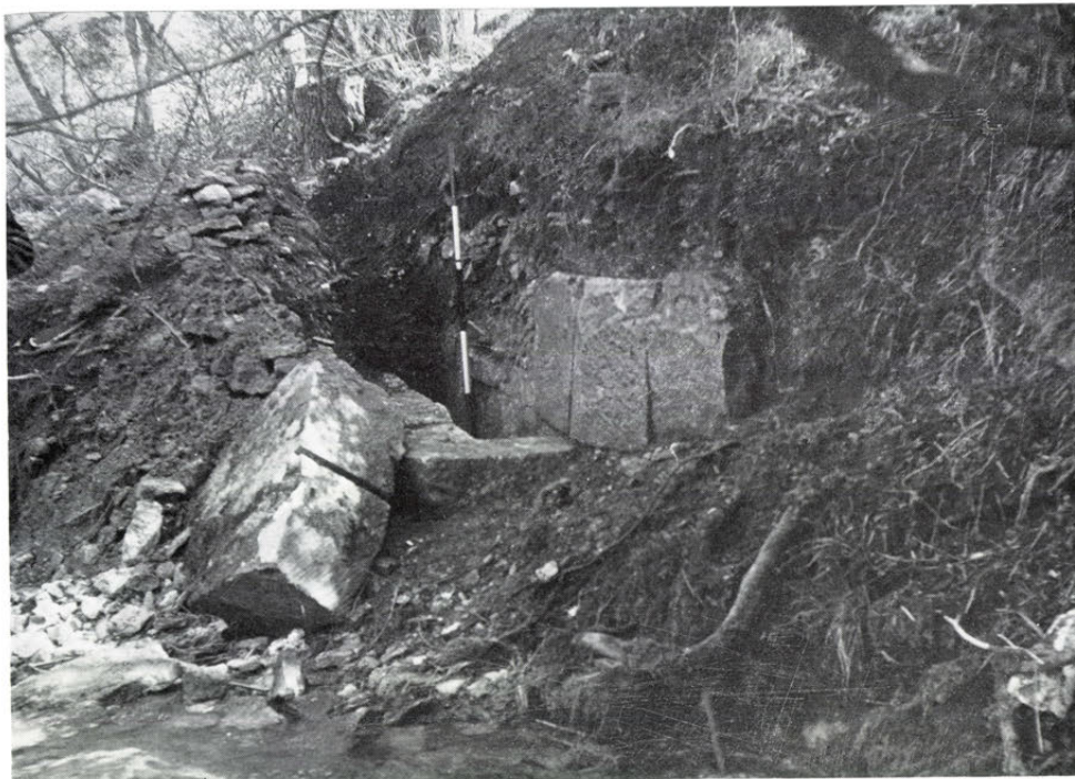
b. Detail of water-wheel housing, looking east. The slot for the sluice which controlled the water supply to the water-wheel may be seen on the side stone blocks (the left-hand block has fallen from its original position)
