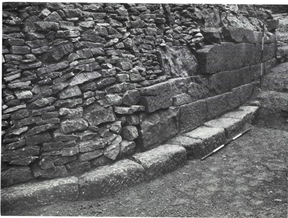
b. North face of rusticated second-phase octagonal podium wall of temple, looking west. The dry-stone walling has been inserted to protect the upper floor levels of the temple
