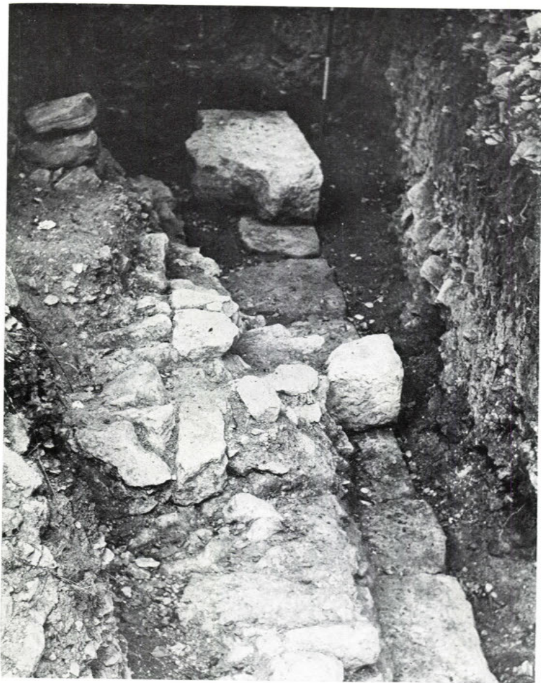
a. Building VII. North riverside wall, looking west, with large stone pier at north-west corner of building
