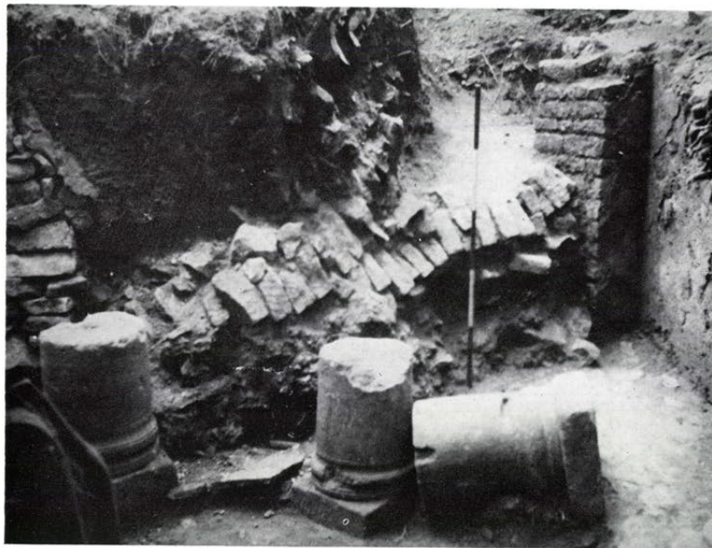
a. Central area of third-phase octagonal shrine, looking south. The collapsed groin of the vaulting is shown lying against the radial wall with column bases as found
