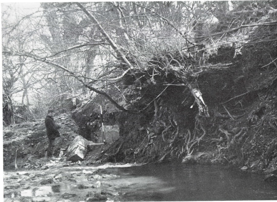
a. The water-wheel housing at the east (downstream) end of the Nettleton settlement looking east
