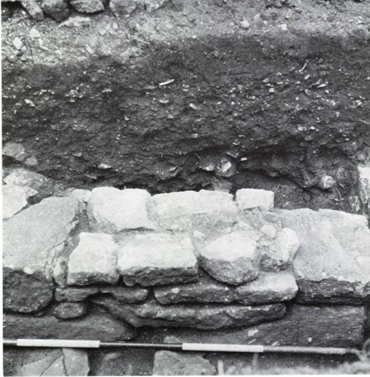
a. Building IX. Blocked doorway in partition wall
