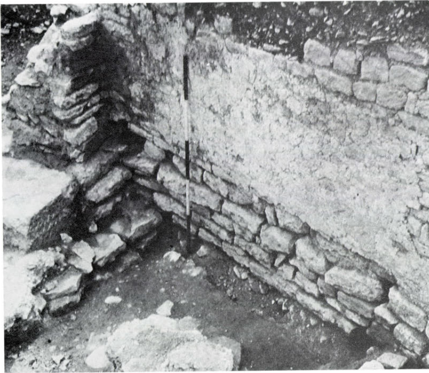
a. Eastern entrance sector of third-phase octagonal temple, showing junction of later radial wall and octagonal wall with entrance pier base
