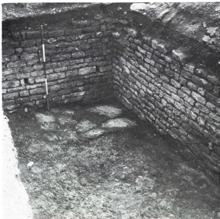
b. Building XIII. Cellar or strong-room looking east
