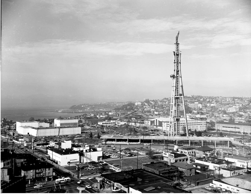
FIGURE 15.1 Construction of the Space Needle and Coliseum (later KeyArena and ultimately Climate Pledge Arena) in 1961. The pyramid shape of the arena roof's supporting structure can be seen near the center of the photo. ("Century 21 from top of the Grosvenor House" courtesy of the Seattle Municipal Archives, item number 165665)
