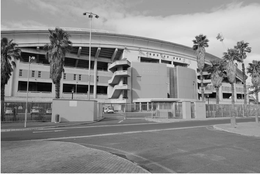
FIGURE 11.2 Athlone Stadium. (Courtesy of the City of Cape Town)
