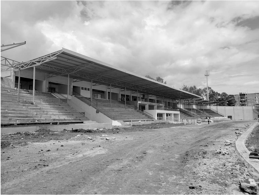
FIGURE 13.3 Interior of Kirigiti Stadium, under construction in January 2022
