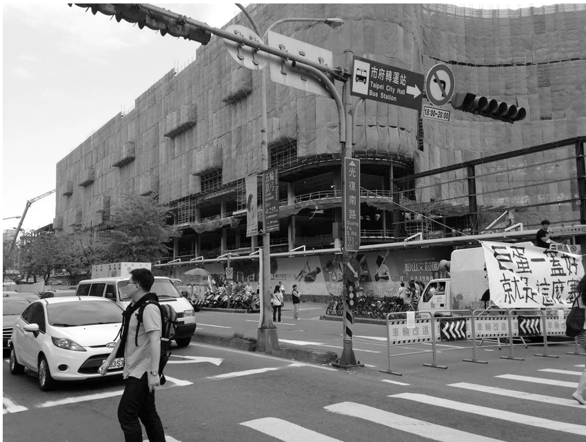
FIGURE 14.2 Construction of Taipei Dome Complex in April 2015. During this time, civic organizations staged a protest, legally closing one-way lanes on Guangfu South Road to simulate traffic congestion during events at the stadium. The banner reads, “Once the domed stadium is completed, this area will experience bumper-to-bumper traffic”
