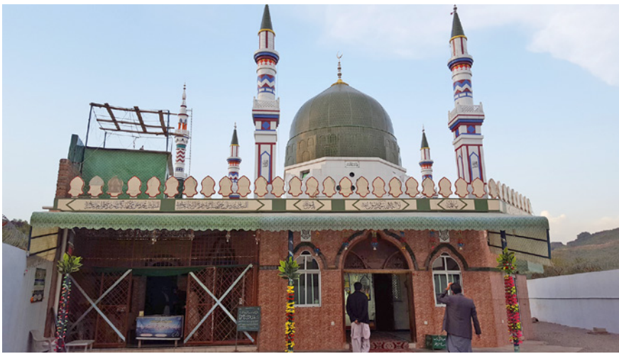
FIGURE 10.2 Qadri's shrine under construction PHOTO: ANONYMOUS, MARCH 2018
