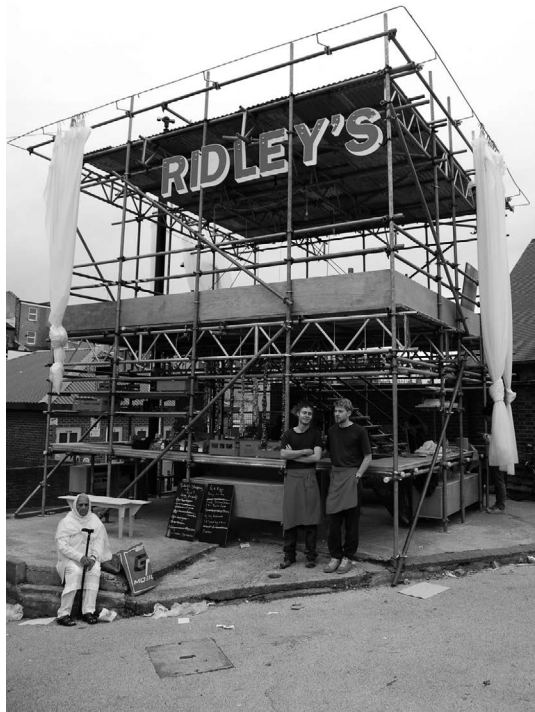
FIGURE 4.9 Dalston: Ridley's Restaurant.
