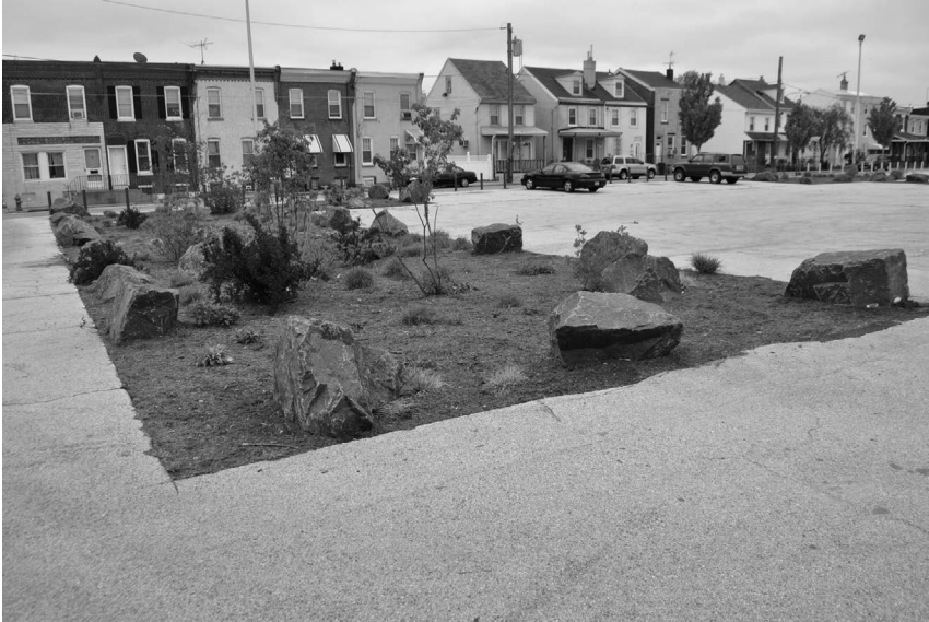
FIGURE 5.9 Philadelphia: rain garden at Eadom Street (parking lot depaved by the Philadelphia Water Department).
