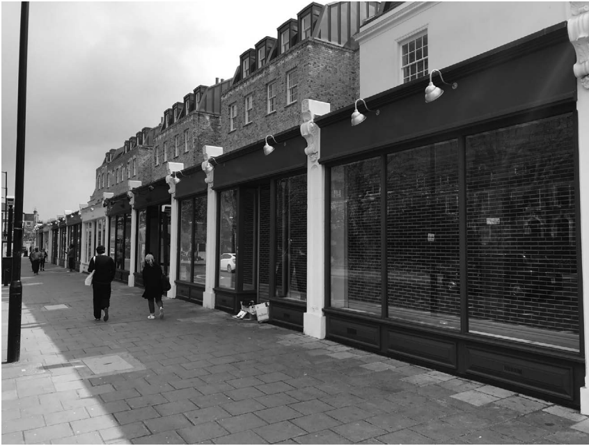
FIGURE 3.5 Dalston; rebuilt facade in Dalston Lane Terrace with codified shopfronts.
