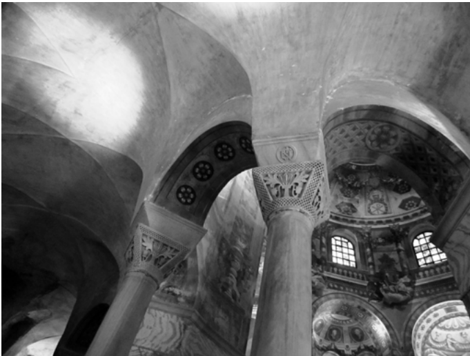
Fig. 13: San Vitale, galleries (photo Baldini).
