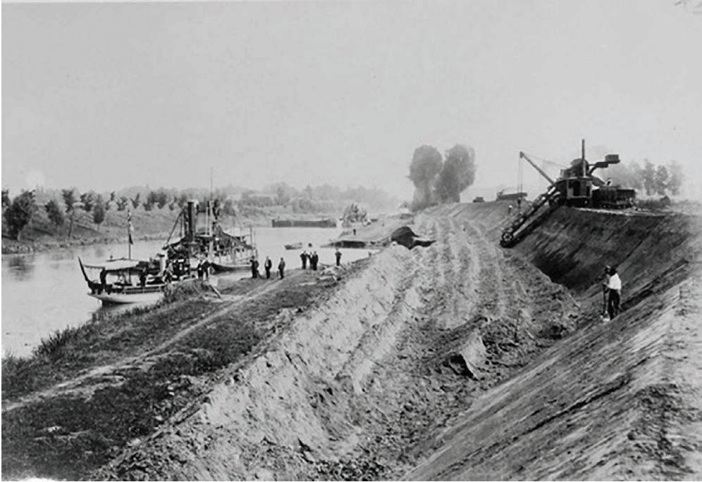
Figure 2.2.8 Construction of the first section of the Maritime Canal (photograph dated 17 July 1901).
