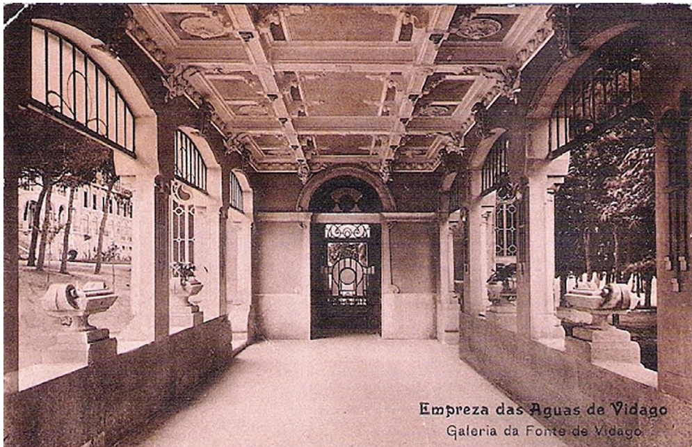
Figure 1.1.7 A reinforced concrete gallery ceiling in the bath house of Hotel Palace do Vidago designed by architect António Rodrigues da Silva Júnior and built by Empreza Construtora do Porto, from 1908 to 1910.
