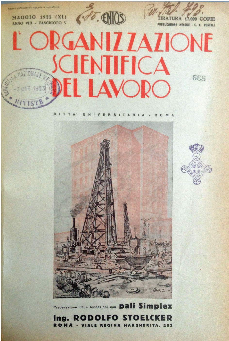
Figure 2.3.19 Pile driving structure used by Stoelcker for the construction site of the University City of Rome.
