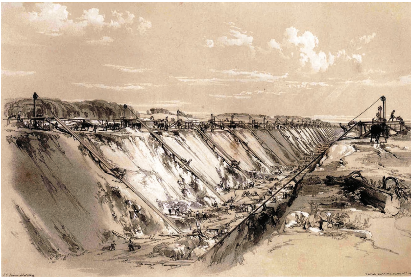
Figure 2.1.13 Tring Cutting on the London and Birmingham; the contractor Thomas Townshend had 40 years' experience in construction (Bourne & Britton 1839).
