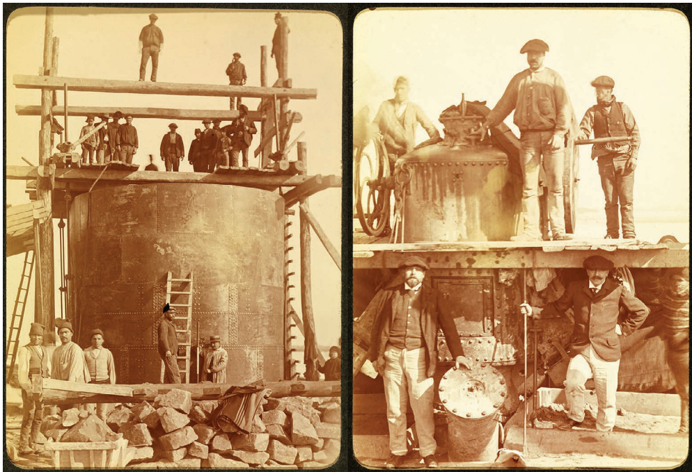
Figure 1.1.2 Left: Steel pneumatic (compressed-air) caisson for the foundation of one of the Rainha D. Amélia bridge piers (1904) to be filled with plain concrete. Right: Air lock used by staff to enter and exit the caisson.
