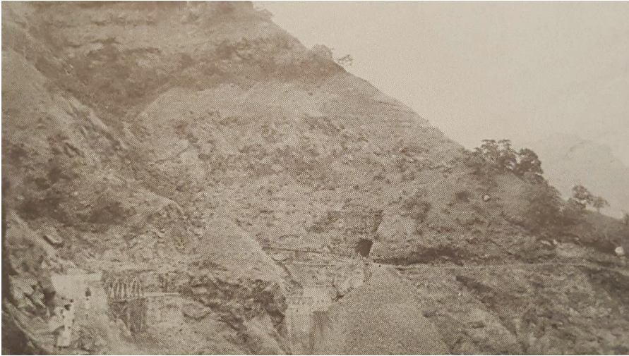
Figure 2.1.28 Bhore Ghat incline on the Great Indian Peninsula Railway, contractors Solomon and Alice Tredwell.
