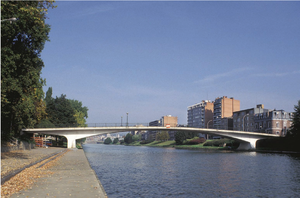
Figure 1.6.7 The Mativa footbridge (1905) in Liège.
