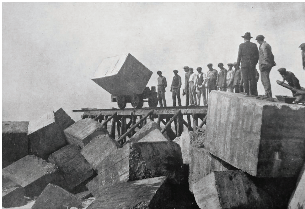
Figure 1.1.11 Concrete blocks in jetty construction for Figueira da Foz harbour with the Portuguese Portland cement, Liz brand.
