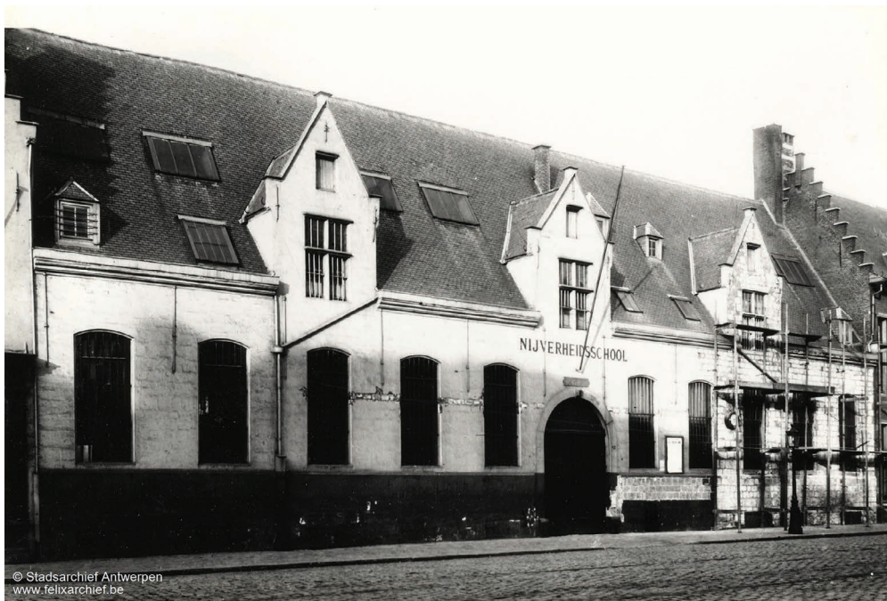
Figure 2.4.4 Façade of the former Nijverheidsschool at Paardenmarkt Antwerp, circa 1925.
