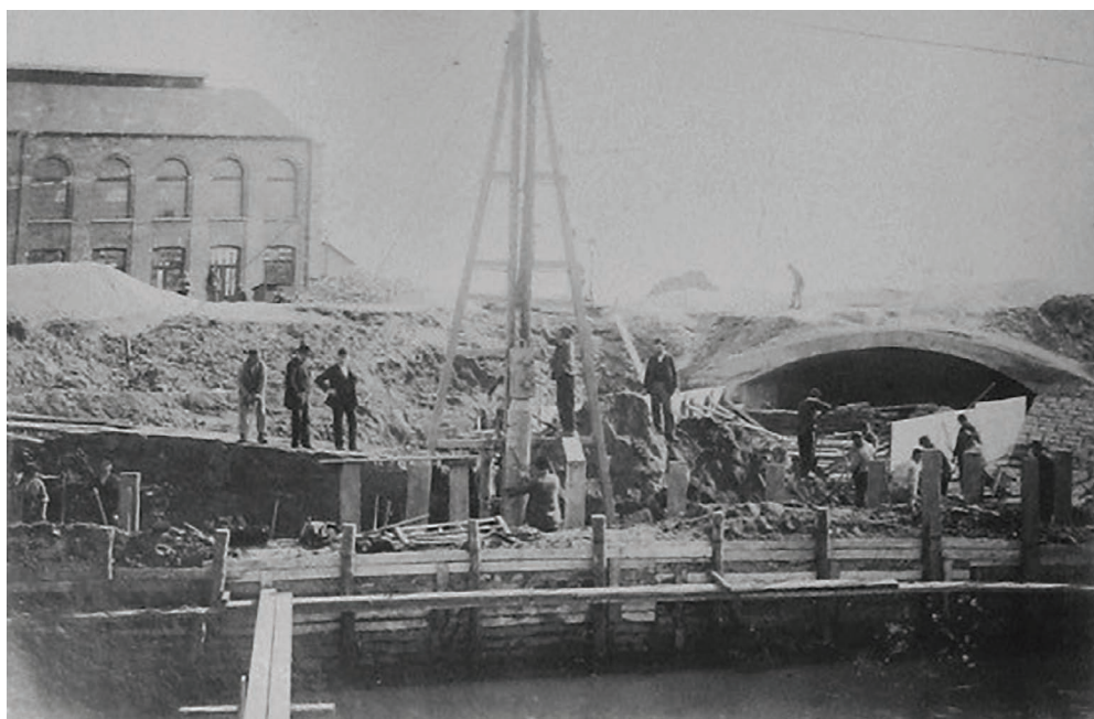
Figure 2.2.7 Construction of the canal tunnel collecting the Maelbeek stream in Schaerbeek, 1894–1895. Note the unreinforced 90-cm-thick concrete vaulted roof of the sewer and the driving of timber piles.
