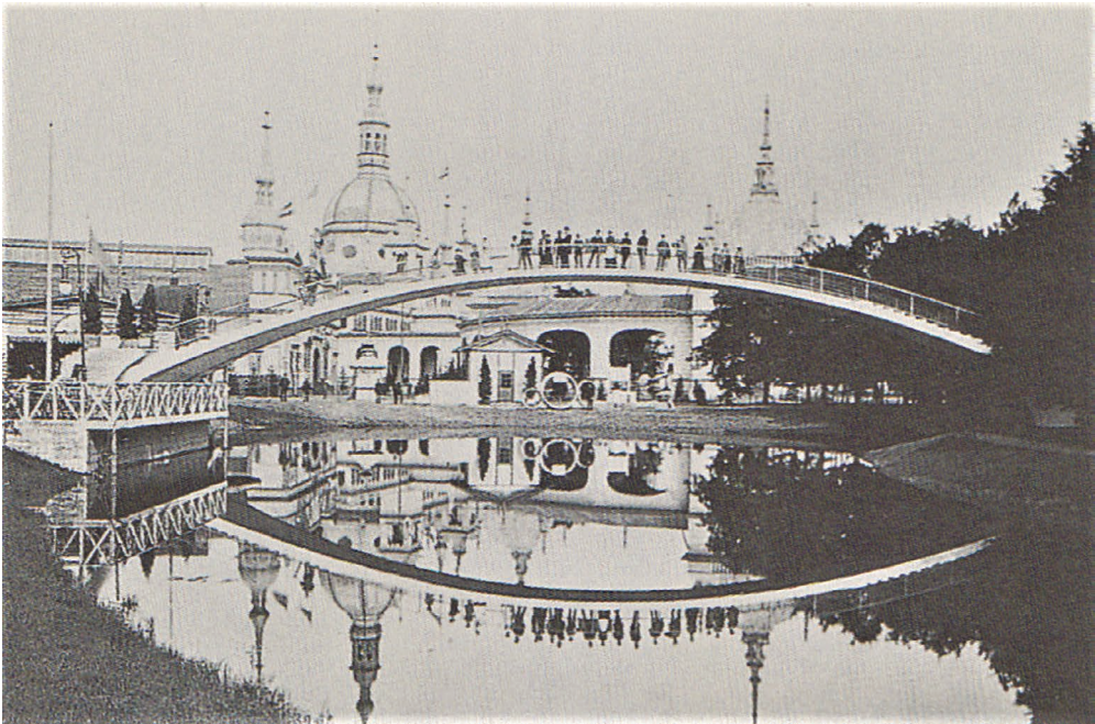
Figure 1.5.4 Reinforced concrete pedestrian bridge built for the Expo in Bremen, Germany. Design: Mathias Koenen, 1890. Source: Bosc et al. (2001: 116).
