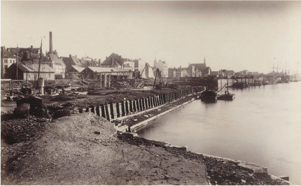
Figure 2.4.3 Rectification of the Scheldt quays to improve port functionality by contractor Couvreur & Hersent, circa 1880.
