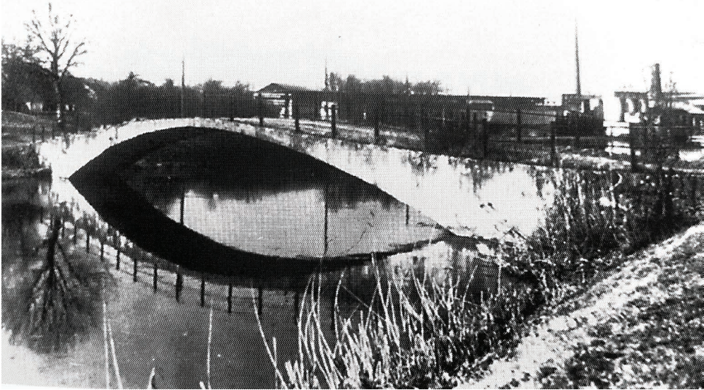
Figure 1.4.3 First reinforced concrete bridge in Switzerland spanning the Aare canal in Wildegg, Actien-Gesellschaft für Monierbauten, 1890.
