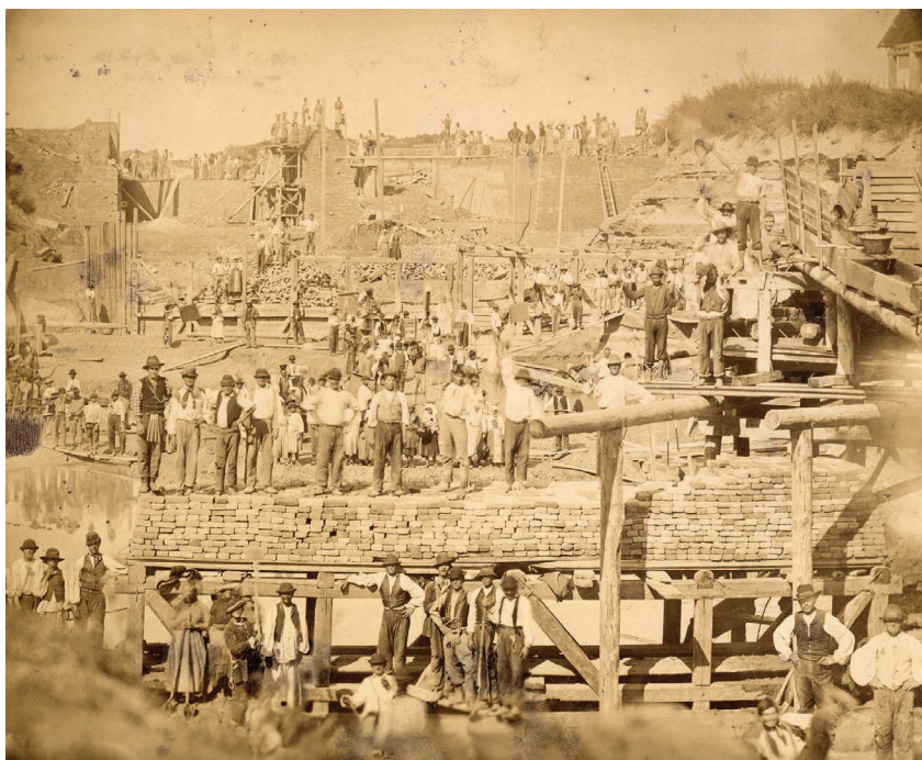
Figure 2.1.18 Work on the Francis Canal in Austria-Hungary in 1874, undertaken by Brassey's Partners George Wythes and J.A. Longridge, photograph.
