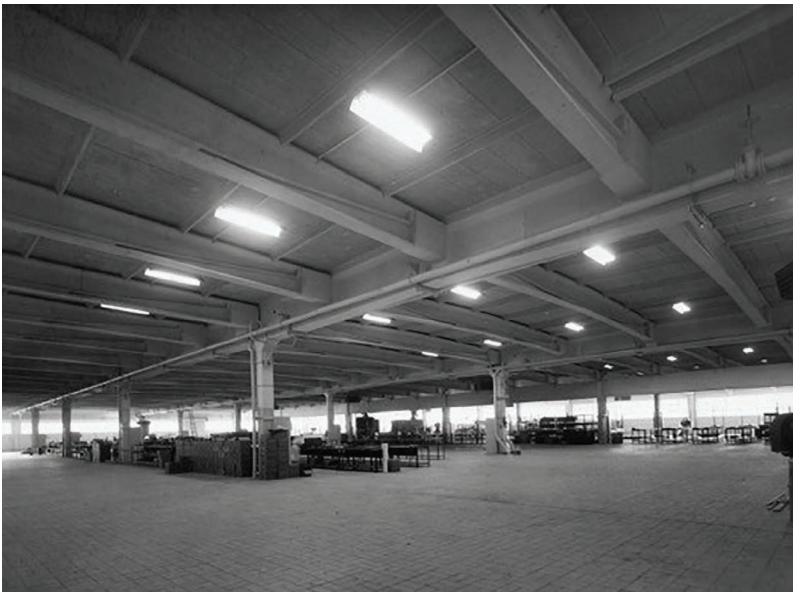
Figure 2.2.14 New workshops for the electronics division of the Ateliers de Constructions Électriques de Charleroi in 1953.
