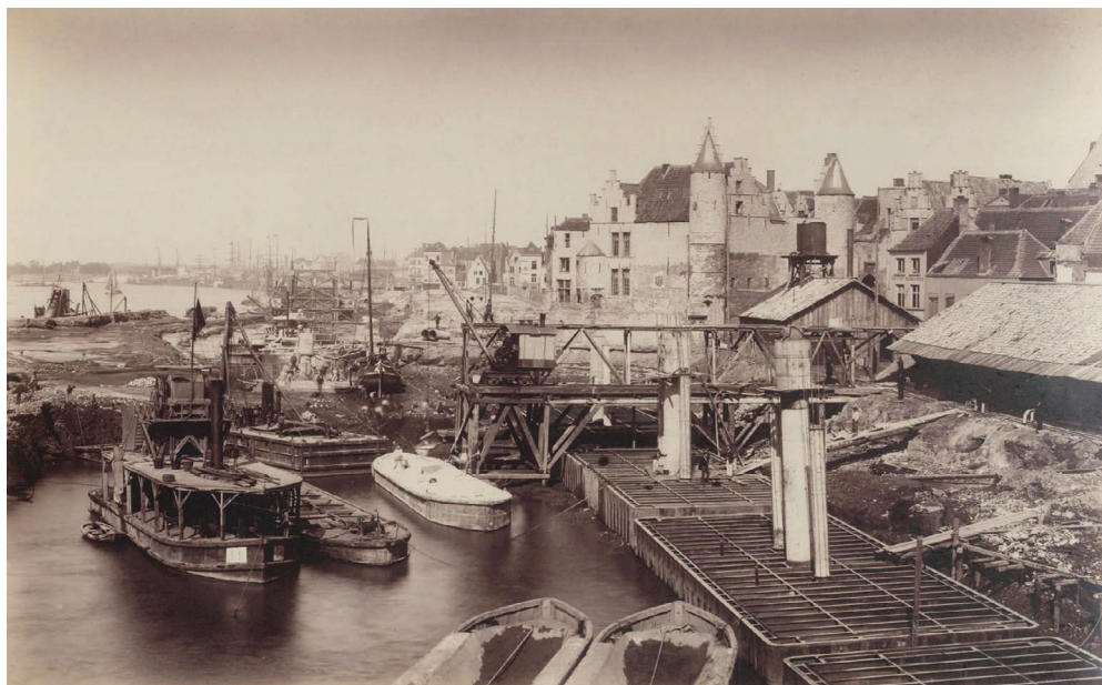
Figure 2.4.2 Demolition of the historic centre and dismantling of “de werf” by contractor Couvreur & Hersent, ca. 1880.
