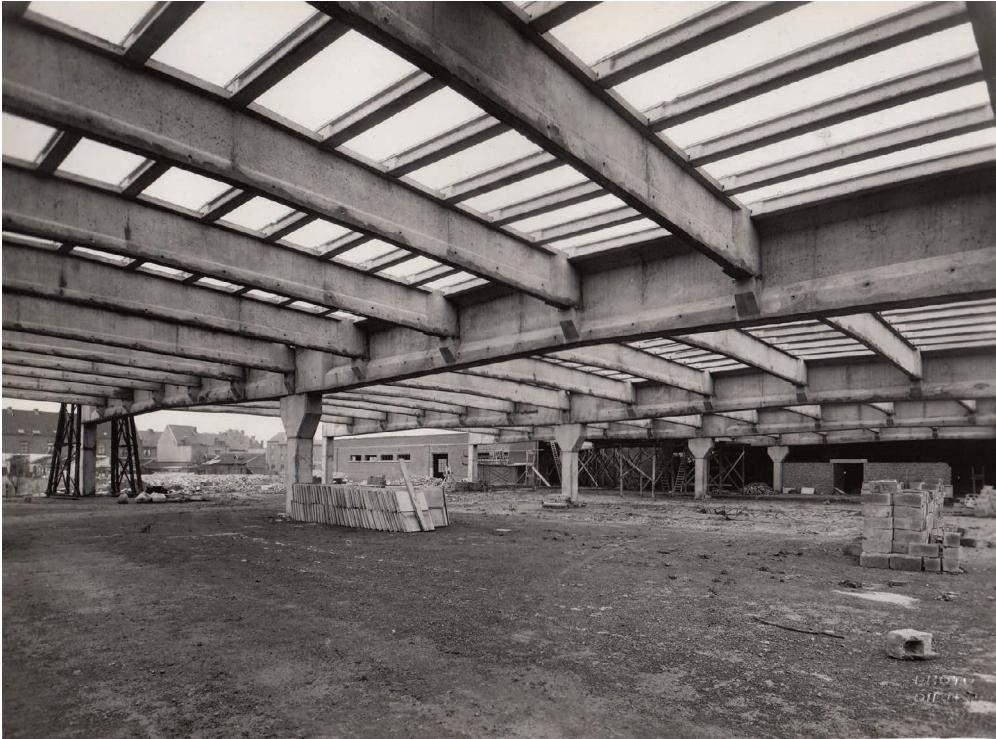
Figure 1.6.11 Construction of the Union Cotonnière mills buildings in 1948.
