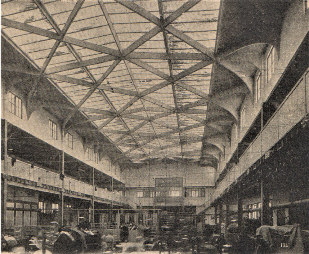
Figure 1.5.5 Factory ceiling, Paris. Design: Cottancin, 1900.
