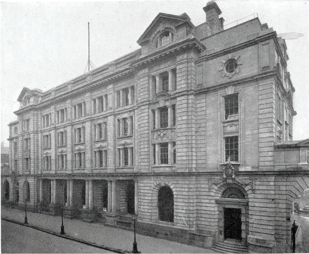
Figure 1.2.15 Tanner's General Post Office building at the date of construction.
