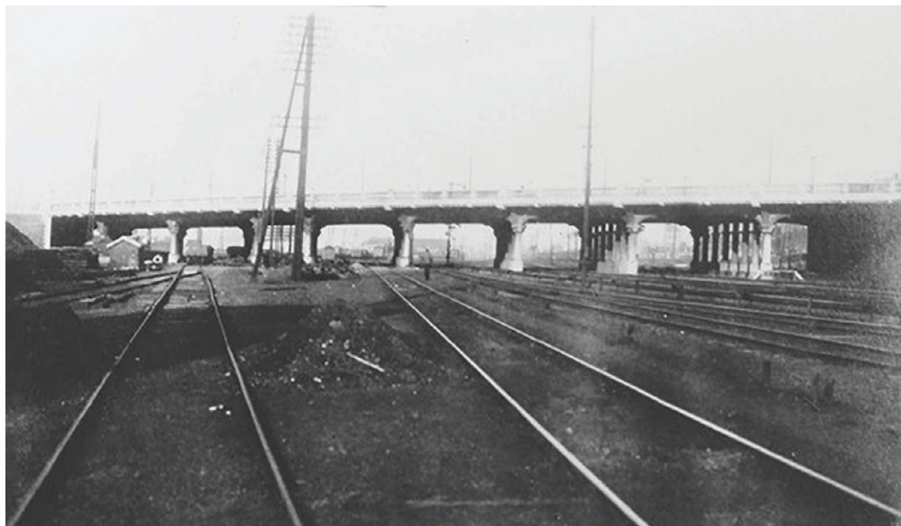
Figure 2.2.9 The Teichman reinforced concrete road bridge built by Armand Blaton over railway lines in Schaerbeek in 1905.
