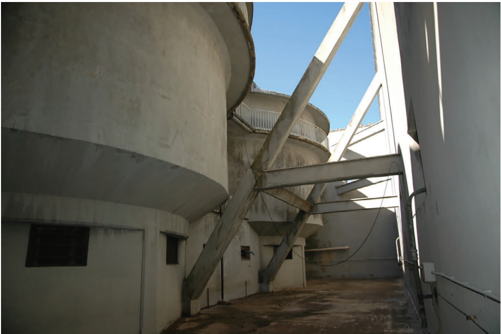
Figure 2.3.17 Interior of the water reservoir on via Eleniana, Rome. The water tanks' profiles near the perimeter wall.
