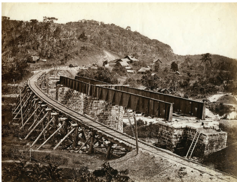
Figure 2.1.12 A typical British railway export: Joannes viaduct on the Bahia and San Francisco Railway under construction by John Watson in 1861; Watson's inability to convert bonds he held on the Mid Wales Railway in the spring of 1866 precipitated the Overend–Gurney crisis of 1866, although he eventually discharged his bankruptcy.
