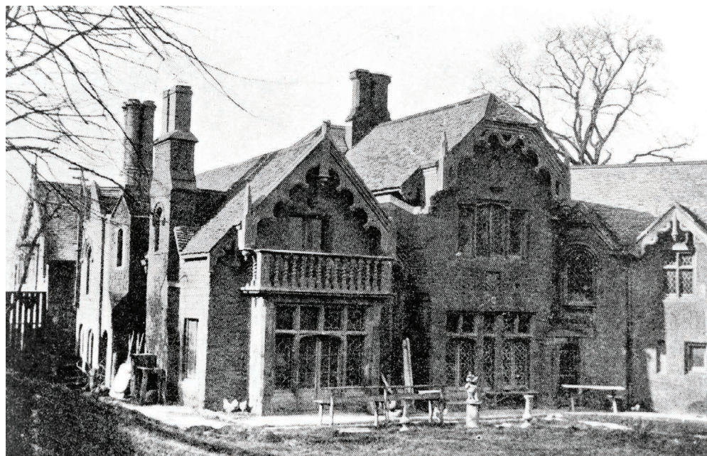
Figure 1.2.2 John Bazley White’s concrete house at Swanscombe, 1835.
