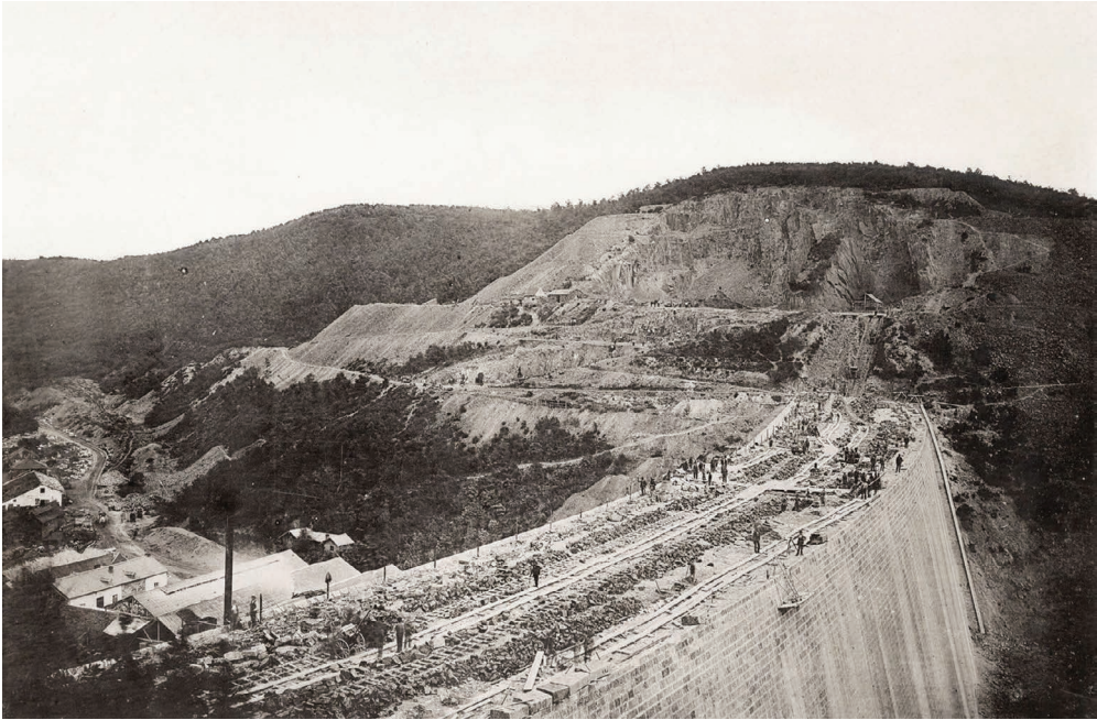
Figure 1.6.1 The Gileppe concrete dam under construction (n.d., before 1878), Jalhay, Belgium. Source: Royal Library of Belgium (S.I 49333).
