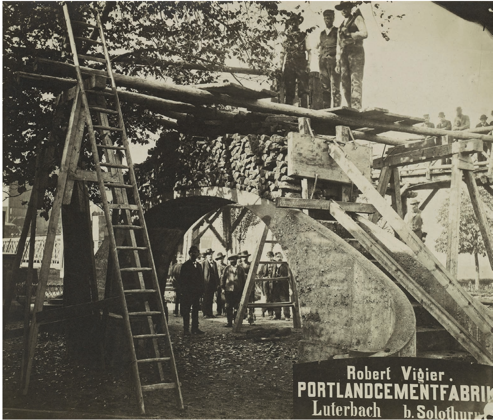
Figure 1.4.5 Concrete bridge by Robert Vigier at the Swiss National Exhibition in Zürich, 1883.
