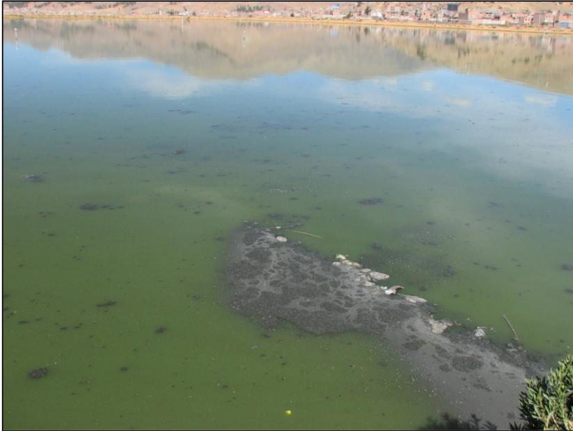
**Figure 5.6** Rising sludge from the anaerobic zone lifted with methane and carbon dioxide bubbles. This facultative pond had excessive sludge accumulation after more than 20 years of operation without sludge removal. In spite of the accumulation, the aerobic zone is still functioning well as seen by the bright green color. Unless the pond is desludged, the rising sludge will eventually cover the surface and the pond will turn anaerobic throughout its depth (Figure 5.7; Puno, Peru).
