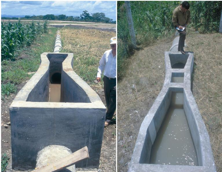
**Figure 4.13** Examples of Parshall flumes that never should have been built. The dimensions are wrong, the construction is poor, and there is no headloss through the structure. For these reasons, pre-fabricated Parshall flumes that have certified calibration should always be used (left photo: Catacamas, Honduras; right photo: Villanueva, Honduras).
