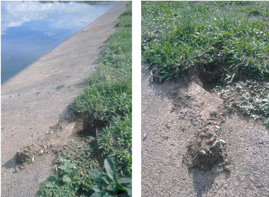
**Figure 10.11** Turtle excavations behind the revetment in a secondary facultative pond. Turtles can burrow behind and under geomembrane liners and the revetment to deposit their eggs. The operator should monitor the condition of a liner and revetment routinely when there are high turtle populations in the ponds (Danlí, Honduras).
