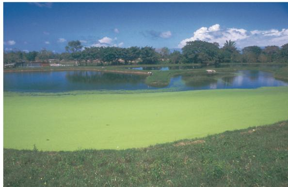
**Figure 10.8** A common example of duckweed, carried by the wind or by birds, that has partially covered the surface of a maturation pond. The operator should remove the duckweed as soon as possible before the pond is entirely covered. Domestic ducks rapidly eat duckweed and a few can be brought to a heavily covered pond to aid in its removal (Tela, Honduras).
