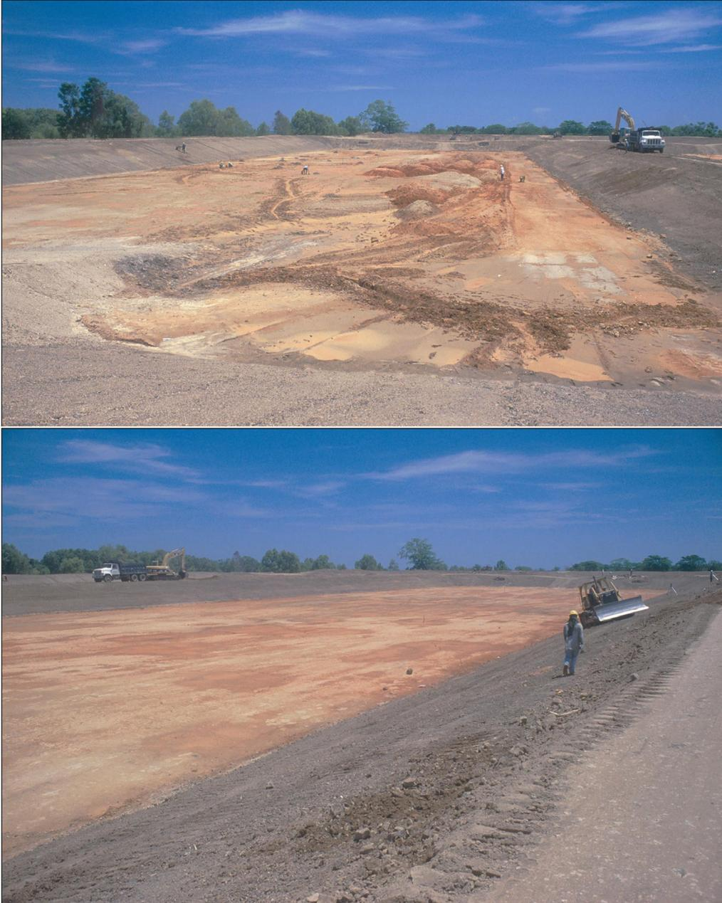
**Figure 9.5** Impermeabilization of ponds with clay which is essential to maintain the water balance and avoid excessive infiltration, with the possible contamination of the groundwater. The clay should be layered with a total thickness of at least 5–10 cm, and covered with a layer of soil to protect it. In this example, the contractor did not put clay on the interior slopes and the pond had excessive infiltration as seen in [Figure 9.4](#) (La Ceiba, Honduras).
