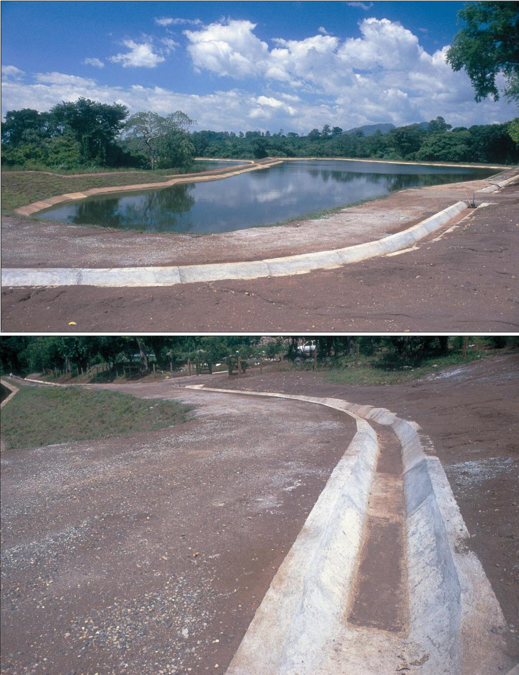
**Figure 9.2** A well-designed and constructed stormwater diversion channel. If the location of the pond system is downstream of stormwater runoff, channels must be used to divert the runoff to avoid erosion of the interior embankment slopes (see [Figure 9.3](#)), and the input of non-wastewater suspended solids is carried by the runoff (Santa Cruz de Yojoa, Honduras).
