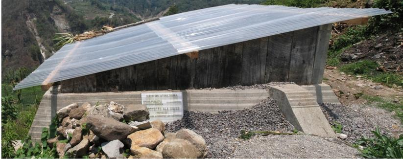
**Figure 8.8** The existing reservoir at the San Antonio, Sololá wastewater reuse project has an estimated maximum volume of 50 m<sup>3</sup> and was designed for a pilot irrigation project of 1.84 ha.
