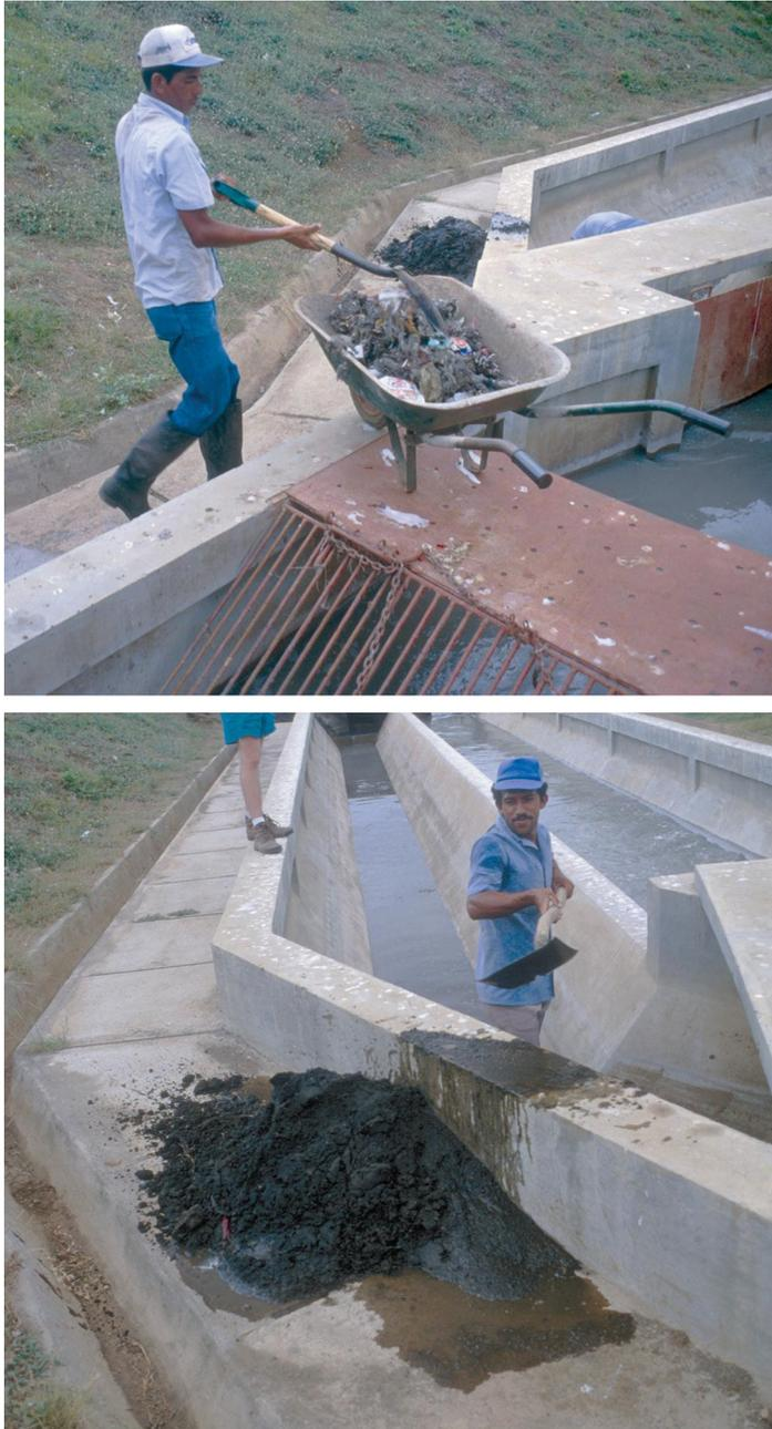
**Figure 10.1** In preliminary treatment, the operator's responsibility is to clean the bar screen daily, and the grit chamber when needed – typically once a week in small systems. It is essential to agitate the settled solids in operating grit chamber on a daily basis so that entrapped organic solids escape to the downstream pond, and inorganic solids remain in the channel. The solids from the bar screen and grit chamber should be buried and covered on a daily basis (Leon, Nicaragua).
