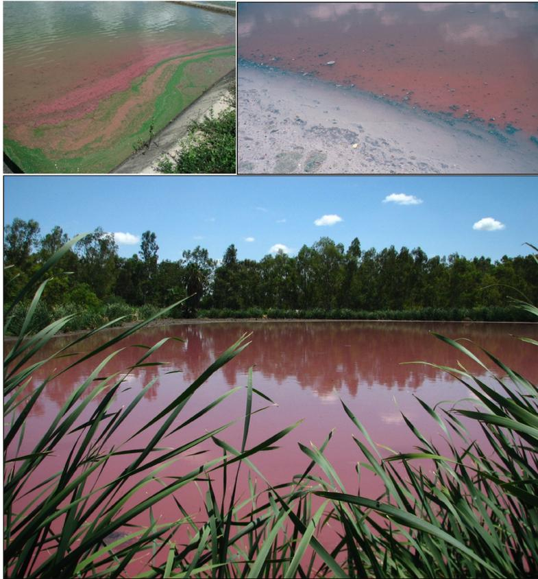
**Figure 5.8** Examples of reddish coloration in facultative ponds as a result of anoxygenic photosynthesis by the purple and green sulfur bacteria. The top left photo is the dead space in a corner of an otherwise well-functioning pond. The top right photo is a highly overloaded pond converting to an anaerobic one. Bottom photo is an overloaded pond (top left: Lagarto, Brazil; top right: Villanueva, Honduras; bottom: Mendoza, Argentina).
