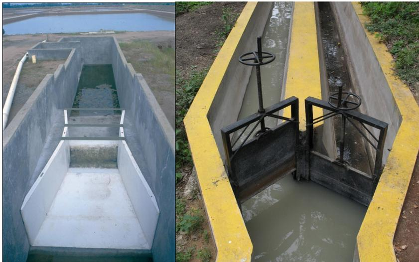
**Figure 9.9** Left: A properly installed, prefabricated Parshall flume used to measure influent flowrates to a facultative pond. Accurate flow measurement is essential for assessment of hydraulic and organic loadings to the pond system. Right: Well-designed and installed sluice gates in a dual channel grit chamber; the gates have metal-to-metal contact that are routinely greased for ease of operation (left photo: El Paraiso, Honduras; right photo: Suchitoto, El Salvador).
