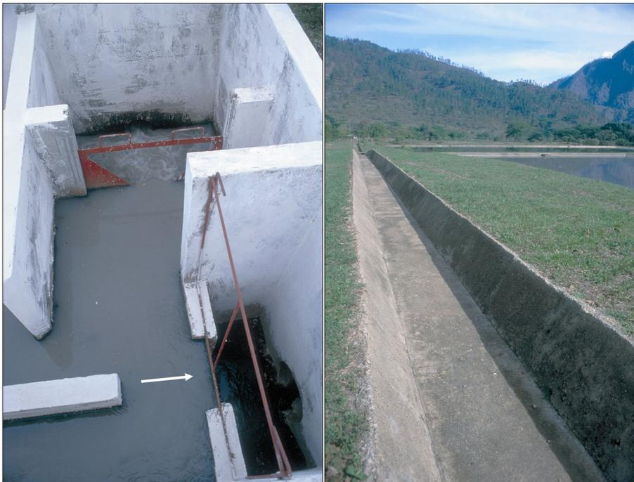
**Figure 9.24** Examples of overflow weirs and bypass channels to protect a pond system from hydraulic overloads during storms. The weir on the right (arrow) in the left photo can be adjusted by the operator when required; when the water level rises above normal during storm events, the excess flow is discharged into the bypass channel. (left photo: Granada, Nicaragua; right photo: Danlí, Honduras).
