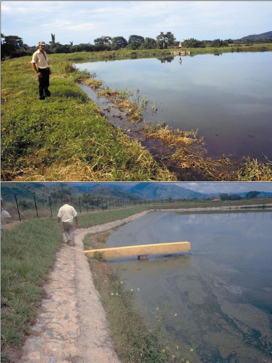
**Figure 9.26** In the photo above (Tela, Honduras), the facultative pond has serious problems with the growth of aquatic plants at the shoreline due to lack of a revetment. In the photo below (Catacamas, Honduras), the poor construction of the revetment (note the contour lines at the water level) with insufficient freeboard does not prevent the growth of aquatic plants.
