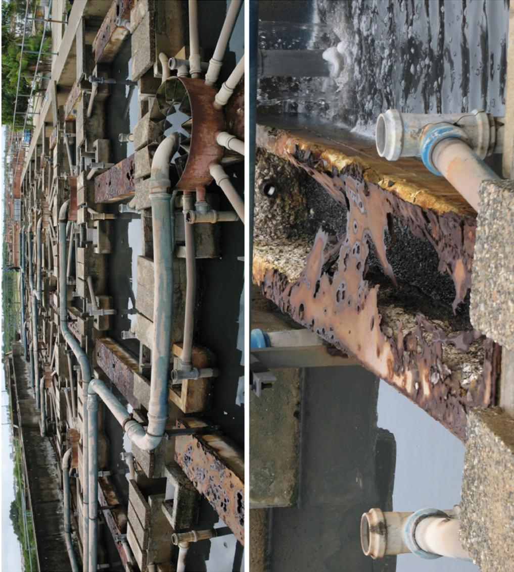
**Figure 2.14** Serious corrosion problems can arise with the production of  $\text{H}_2\text{S}$  and  $\text{H}_2\text{SO}_4$  in UASBs as shown in this unit in Aracaju, Brazil. Raw wastewater monitoring for sulfate concentrations, and the use of corrosion-resistant materials throughout the UASB, must be specified by design engineers to avoid these problems.
