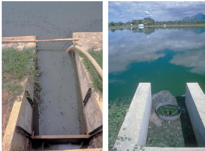
**Figure 10.6** Left photo: the outlet of a facultative pond designed with a bottom sluice gate and a rectangular weir did not have the sluice gate in place; as a result, the floating solids were carried out with the effluent over the rectangular weir, and the removal efficiency of fecal coliforms was low (Catacamas, Honduras). Right photo: a circular baffle is used to control the discharge of scum in the effluent of a facultative pond (Chinendega, Nicaragua).
