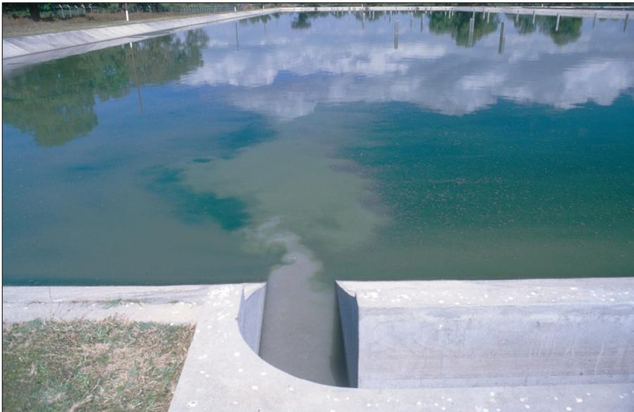
**Figure 9.12** A good example of an inlet structure with open channel that enters this facultative pond at the water level. The raw wastewater plume entering the pond is clearly seen to be approximating plug flow (Granada, Nicaragua).
