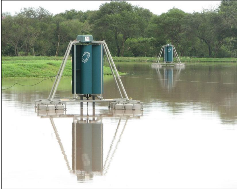
**Figure 5.20** Wind-powered slow mixers in a facultative pond of the sanitation cooperative SAGAUPAC, Santa Cruz, Bolivia. If properly employed, the slow mixers greatly reduces vertical stratification and hydraulic short circuiting.
