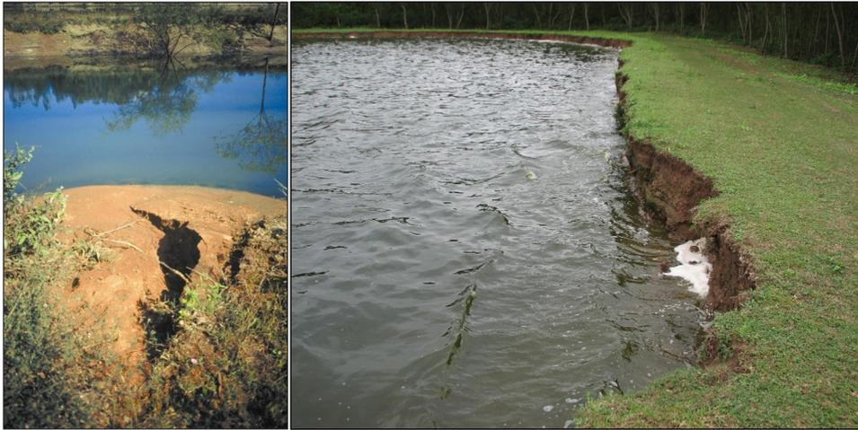
**Figure 9.3** Stormwater runoff has to be controlled to protect the interior embankment slopes of ponds. Left: In this maturation pond, stormwater runoff was not controlled and caused serious erosion to the interior embankment, which did not have protection with a revetment (Zaragoza, El Salvador). Right: Wave action driven by strong winds erodes the unprotected interior embankment of this maturation pond (Santa Cruz, Bolivia).
