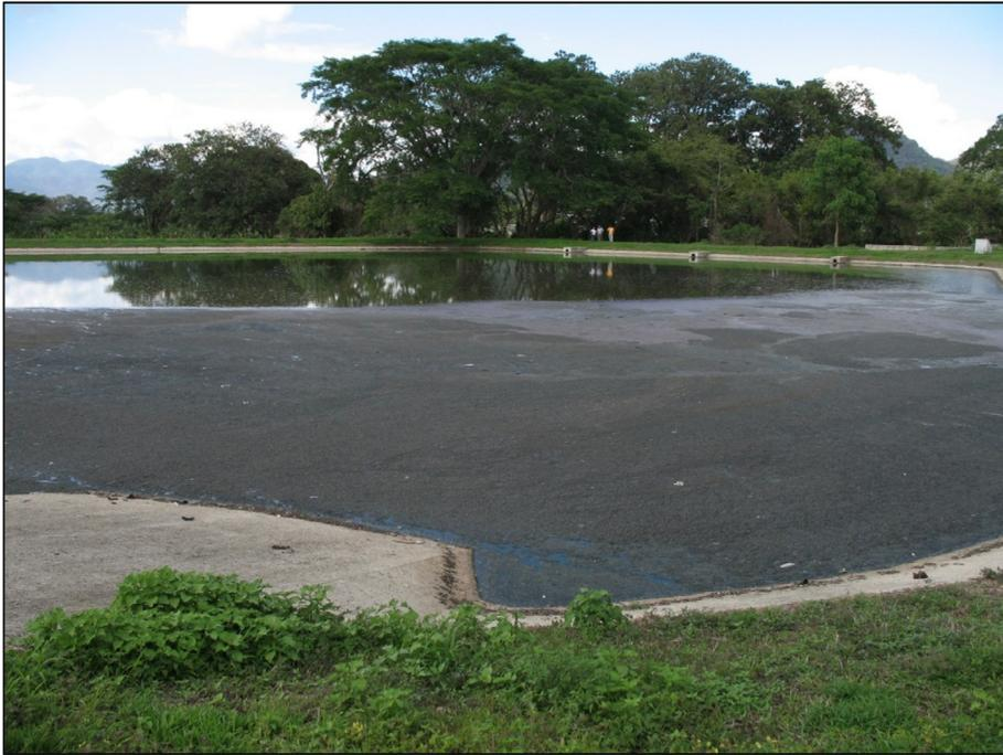
**Figure 5.7** A continuation of the process shown in [Figure 5.6](#). Rising sludge from excessive accumulation is gradually covering a facultative pond. This pond operated for more than 15 years without desludging and is now anaerobic, with the maximum release of methane into the atmosphere (El Paraiso, Honduras).
