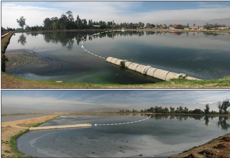
**Figure 5.28** The inlet (top) and outlet (bottom) of facultative pond LP1 (Figure 5.24). The single inlet/outlet locations in a rectangular pond caused significant hydraulic short circuiting with large dead spaces in much of the volume, and sludge accumulation along the shoreline to the left of both the inlet and outlet in the direction of flow. Note the sludge accumulation to the left of the inlet (Albarrancho Wastewater Treatment Plant, Cochabamba, Bolivia).
