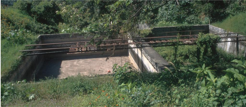
**Figure 2.8** An abandoned activated sludge treatment plant in an urbanization within the city of San Salvador, El Salvador. New developments often require wastewater treatment to be approved, and activated sludge is chosen to save land area for more housing. The cost of operation and need for skilled personnel, however, is normally beyond the resources of the urbanization, and treatment plants like this one quickly fail, if they were ever in operation to begin with.
