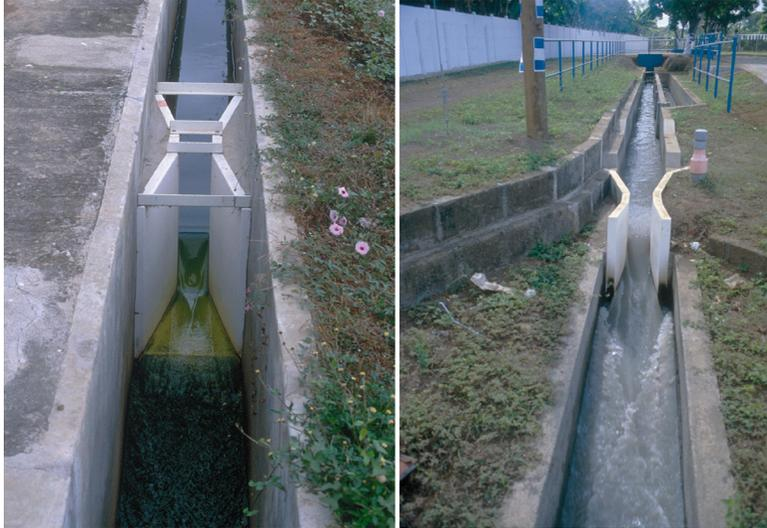
**Figure 4.12** Examples of free-flow Parshall flumes used with horizontal grit chambers. To ensure free flow, the downstream head at the maximum flowrate,  $H_{d,max}$ , must be  $\leq 0.60 H_{max}$ . In the examples above the invert elevations of the downstream canals are much lower than the Parshall flume invert and thus give an added safety factor ( $H_{d,max} \ll 0.60 H_{max}$ ) (left photo: León, Nicaragua; right: Masaya, Nicaragua).
