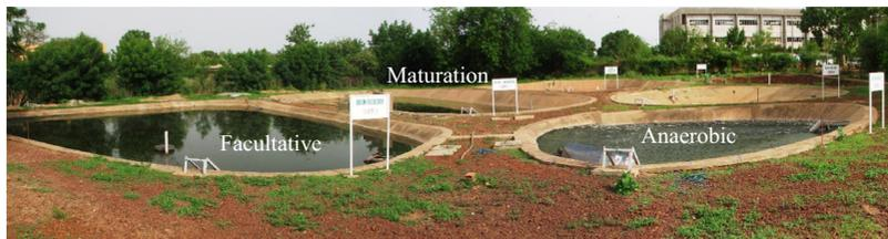
**Figure 1.30** The anaerobic–facultative–maturation waste stabilization pond system at the International Institute for Water and Environmental Engineering (2ie), Ouagadougou, Burkina Faso. The system treated domestic wastewater for a population equivalent of 448 persons, with a mean flowrate of 55 m<sup>3</sup>/d, and a theoretical hydraulic retention time of 18 days.
