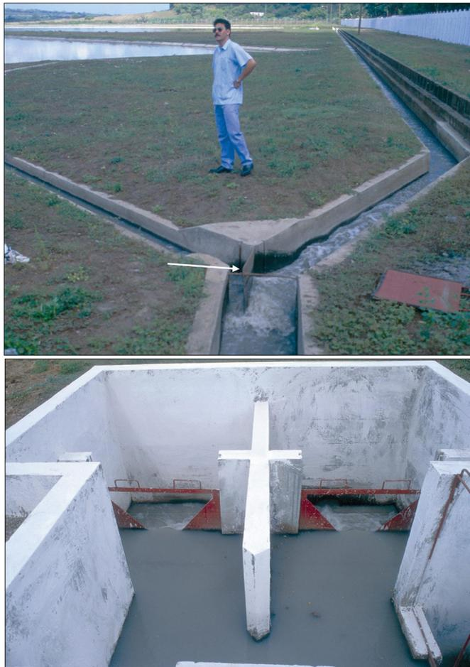
**Figure 9.16** Examples of flow distribution devices between batteries of two facultative ponds in parallel. In the top photo (Masaya, Nicaragua), an adjustable partition is used (arrow). In the bottom photo (Granada, Nicaragua), a fixed partition between ponds in the center is combined with adjustable triangular weirs. The flows to each pond must be monitored to ensure equal distribution.
