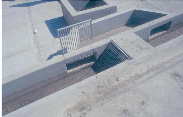
**Figure 4.6** The approach channel to the bar screen should have a bypass as shown above to divert the flow during an emergency when the operator is not available to clean the screen. Note in the photo that the bars are made of aluminum. The influent bar screen should have a drainage platform as shown in [Figure 4.4](#) (Sanarate, Guatemala).
