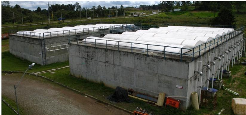
**Figure 2.13** A well-designed and constructed UASB system for a population of 125,000. The methane is flared and not used as an alternative energy source (Rionegro, Colombia).
