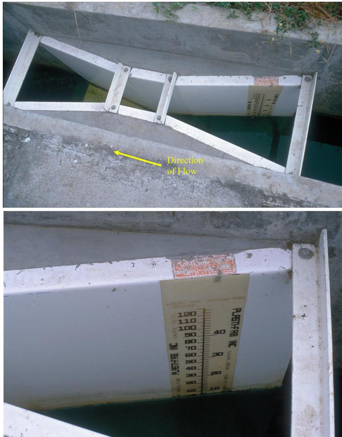
**Figure 4.11** An example of a pre-fabricated Parshall flume installed for a horizontal flow grit chamber. The designer should always specify pre-fabricated and calibrated Parshall flumes in the design to avoid the construction problems shown in Figures 4.13 and 4.14 (Masaya, Nicaragua).
