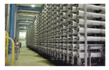
**Figure 1.10** Seawater reverse osmosis membrane filtration installation in Larnaka, Cyprus. The permeate production capacity is  $54,000 \text{ m}^3/\text{day}$ . The total amount of eight-inch diameter membrane elements is 5,800. The plant size can be estimated from the person shown on the left of the figure
