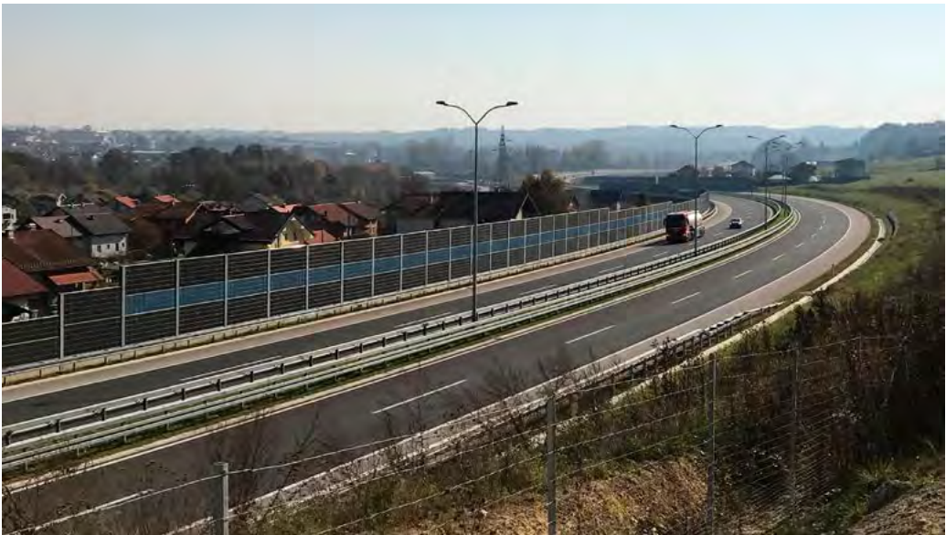
Banja Luka – Doboj Motorway, Republika Srpska, Bosnia and Herzegovina
