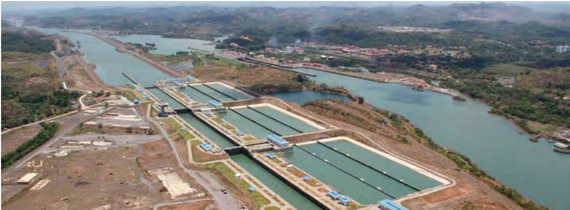
Panama Canal Expansion
