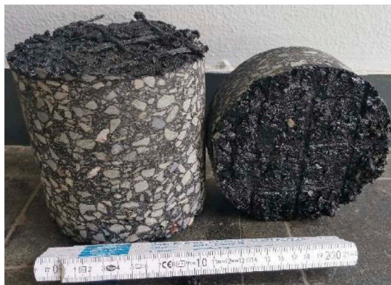
Figure 3. Drill core with reinforcement (after testing).
