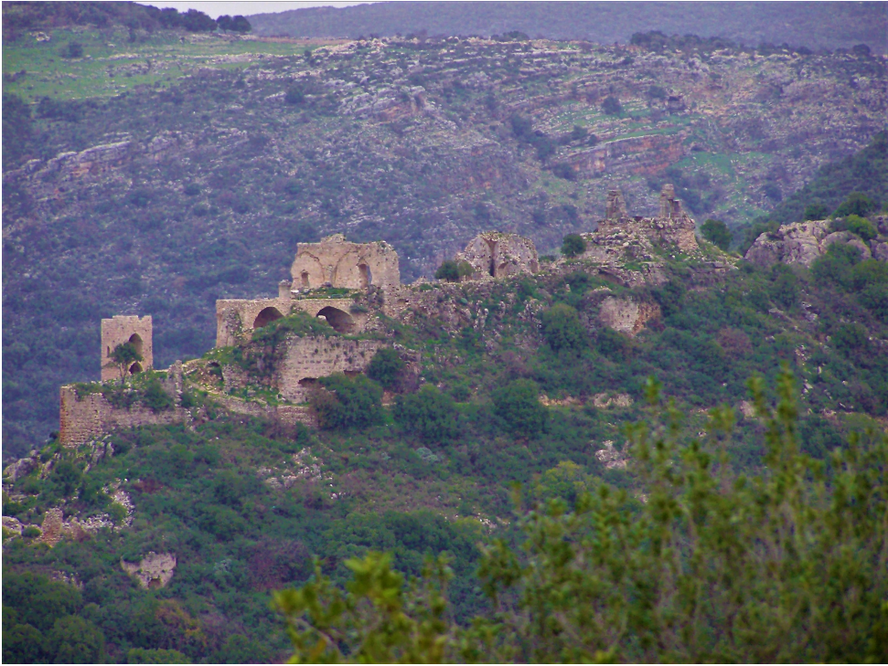
Fig. 1: General view of Montfort Castle in the western Galilee (© Adrian Boas and Rabei Khamisy).
