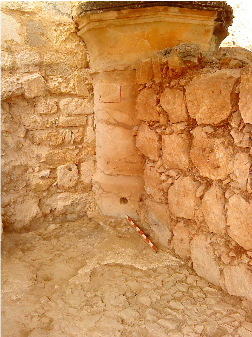
Fig. 12: Temporary support wall in the ruins of the Great Hall (© Adrian Boas and Rabei Khamisy).
