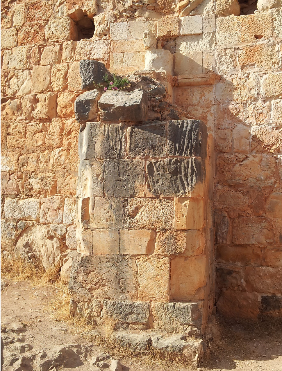
Fig. 16: Strengthening of the domestic ward structure (© Adrian Boas and Rabei Khamisy).
