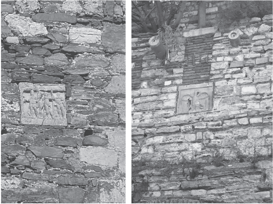
FIGURE 3.18. Building techniques of the city walls in Smederevo and Constantinople. ( Photograph by Jelena Bogdanović )
