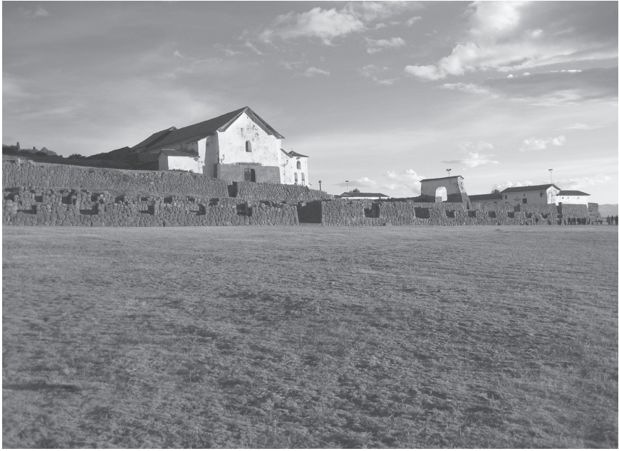
FIGURE 6.7. Chinchoero, Great Plaza with kallanka buildings. (Photograph by Brian Garrett)
