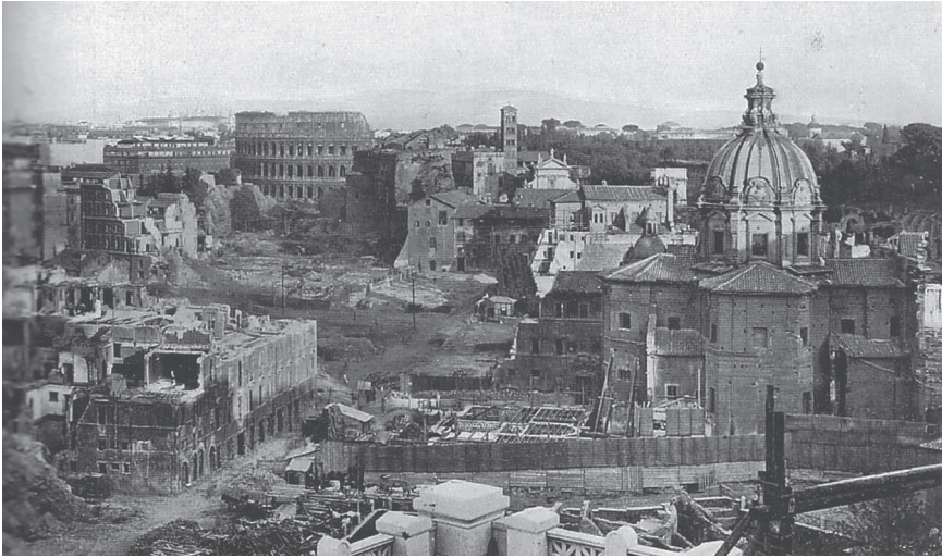
FIGURE 9.2. Demolition underway at the Imperial Fora. (From Capitulum, 1932)
