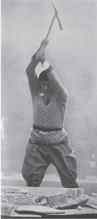
FIGURE 9.6. The first page of the Capitulum article on the inauguration of the demolition at the Mausoleum of Augustus, 1938.
