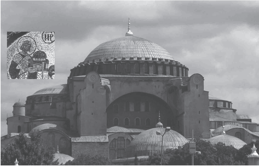
FIGURE 3.4. Church of Hagia Sophia, 532–537, Constantinople, modern Istanbul, Turkey; Anthemius of Tralles and Isidorus of Miletus, architects. Insert: Detail of the golden mosaic above the southwestern entrance of Hagia Sophia, showing Emperor Justinian presenting the church. (Photograph Jelena Bogdanović)
