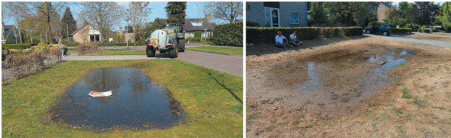
Figure 32.4: Bio swales in wet conditions and after 7 weeks of drought ( https://www.climatecan.org/projects/1114/detail ).
