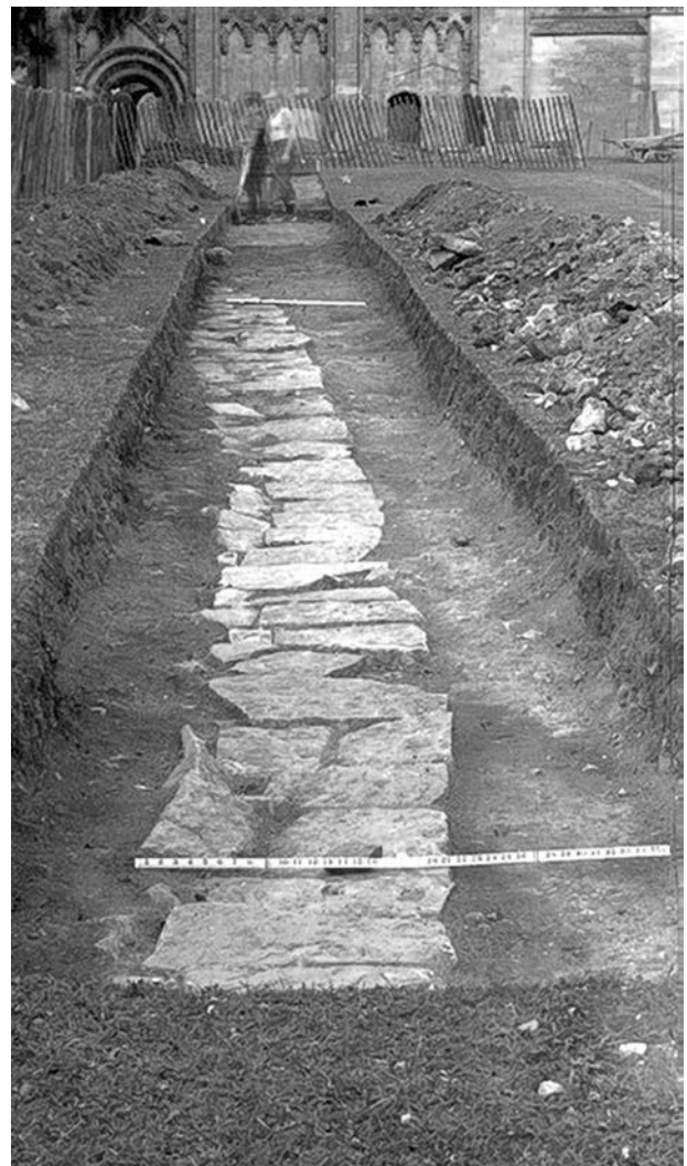
Fig 6.28 Late eighteenth-century wall, looking north (1962 photograph: © EHA)
