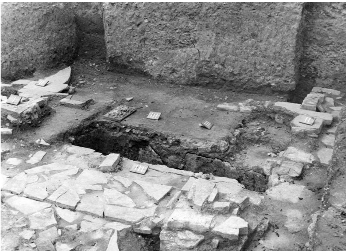
Fig 4.22 Flooring and walls, looking west (1926 photograph: © Glastonbury Abbey)
