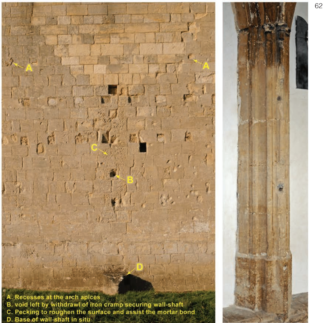
Fig 9.12 Carved stones: (61) '2 inch roll' type mouldings with roof boss (far left), all probably deriving from the vaulting of Abbot Chinnock's cloisters (?after c 1407); (62) scars left on the south elevation of the south nave aisle wall from the erection of the fifteenth-century cloister (left). The rectangular recesses in two regular registers belong to the first post-fire cloister. An analogous campaign in Wells Cathedral's west cloister (from the third quarter of the fifteenth century) also pinned the new wall-shafts to the thirteenth-century wall using lead-grouted iron dog-cramps which have subsequently spalled the stone surface exposing their ends (right) (photos: Jerry Sampson)
