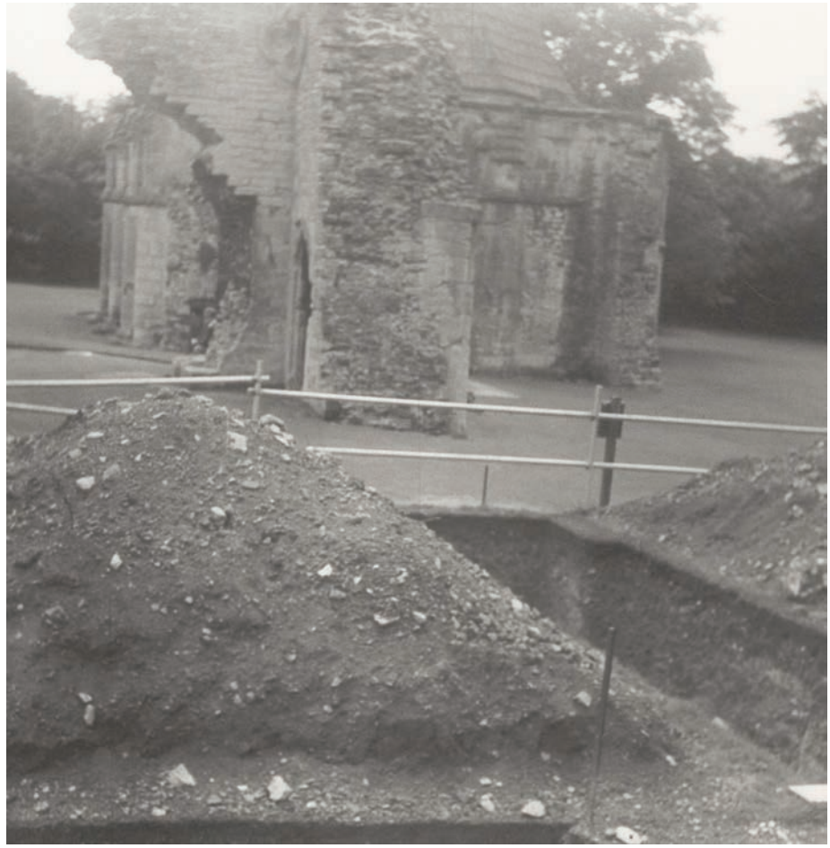
Fig 6.24 Excavations at the north-eastern corner of the hall, looking south-south-west (1978 photograph: © Glastonbury Abbey)
