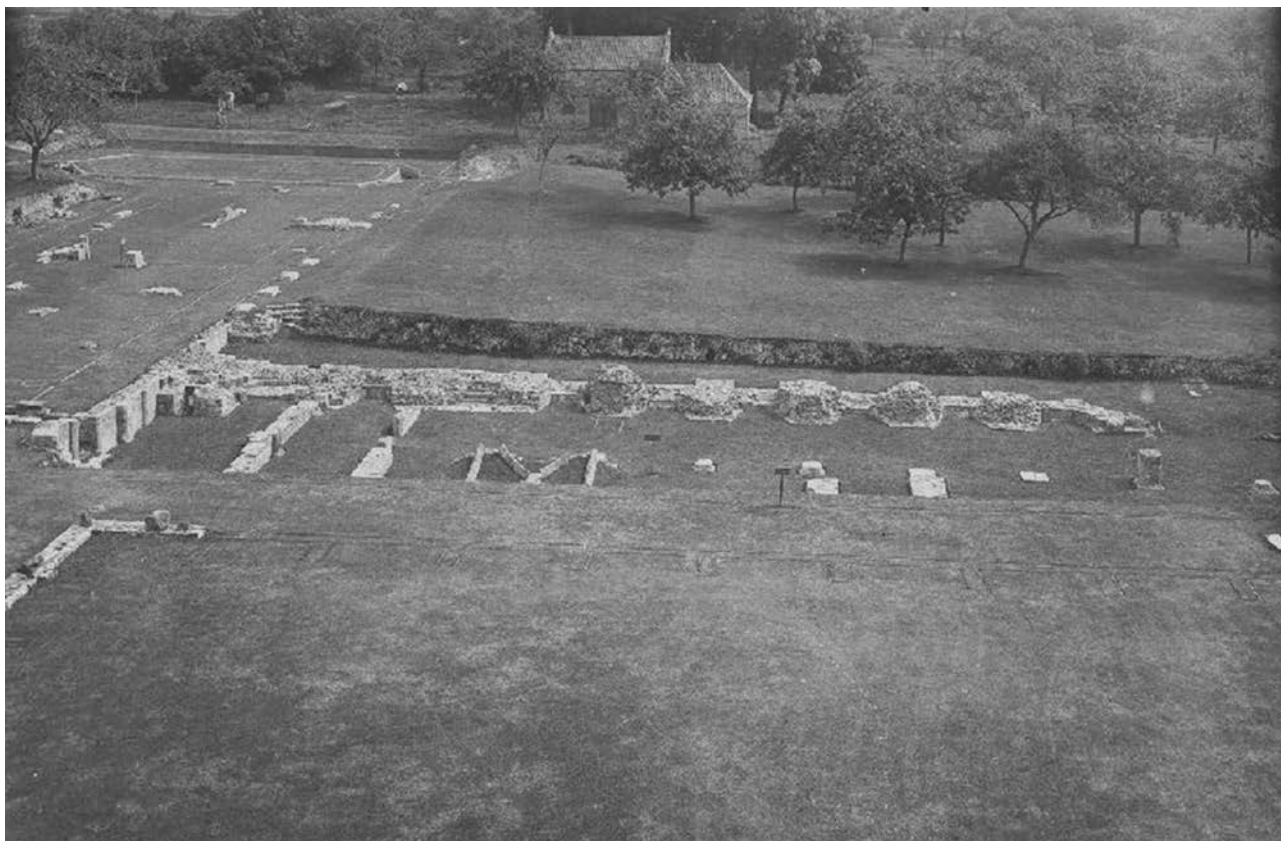
Fig 3.16 1935 photograph showing the refectory and dormitory undercrofts, reredorter and the cider house, looking south (© Glastonbury Abbey)
