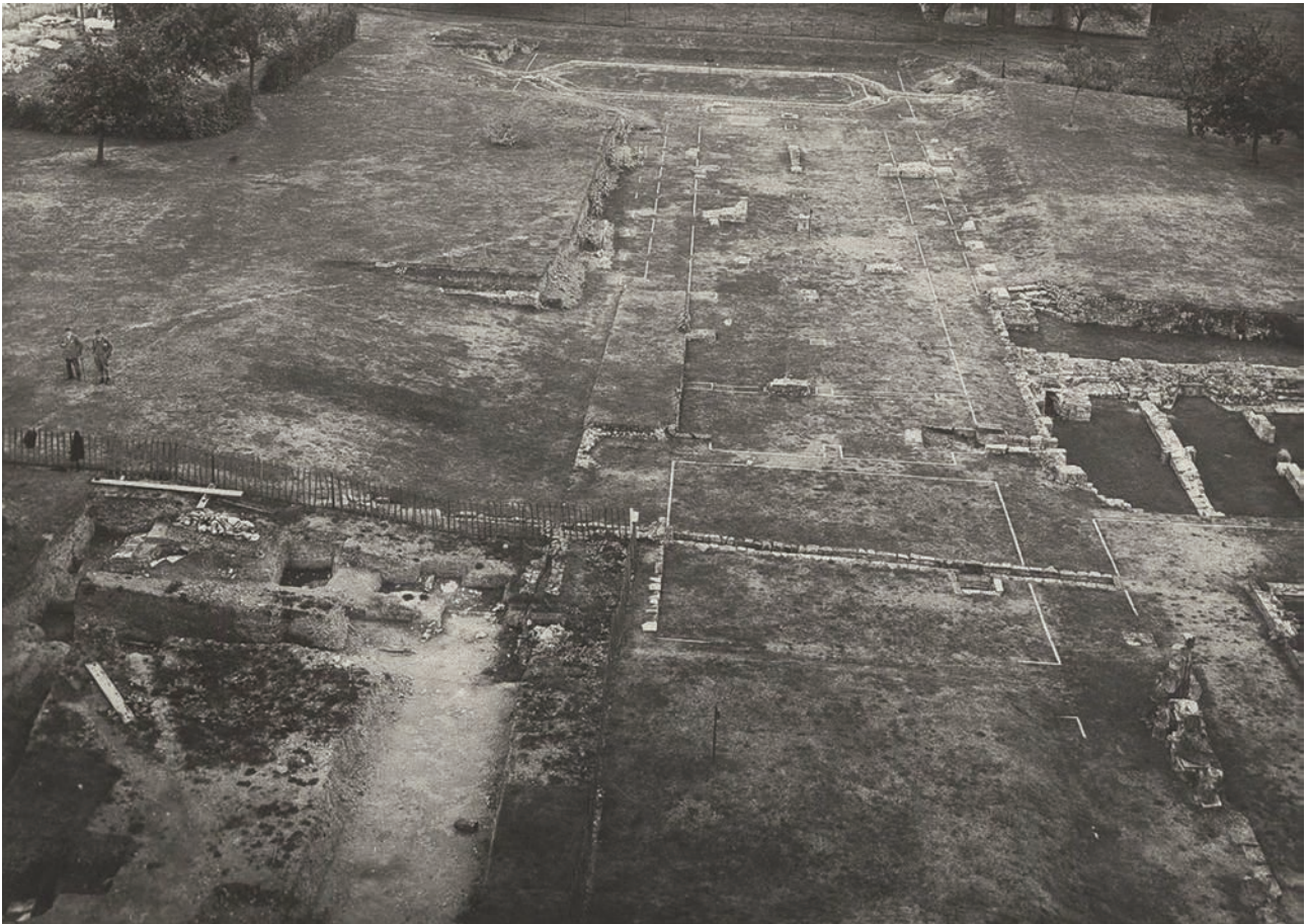
Fig 5.45 Chapter house excavations looking south (1935 photograph: © Glastonbury Abbey)
