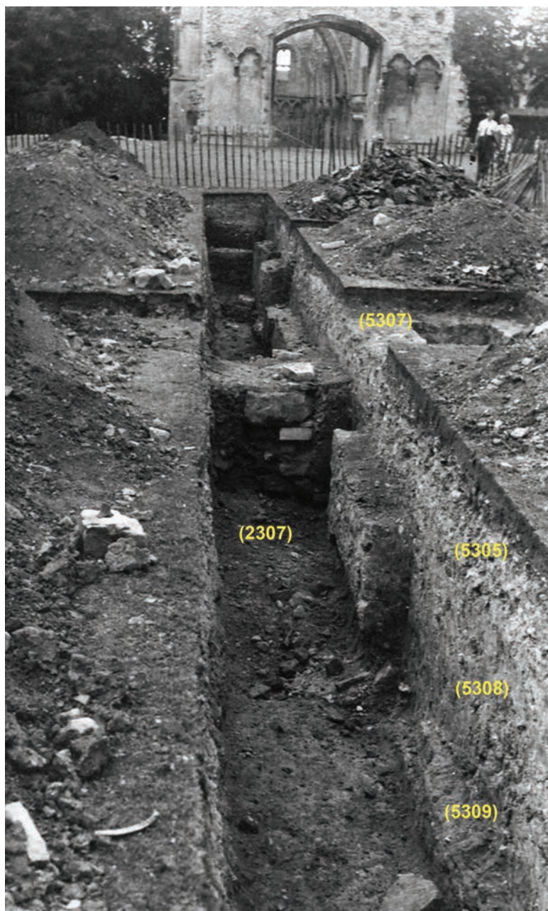
Fig 4.32 Nave trench, looking west (1959 photograph: © EHA)
