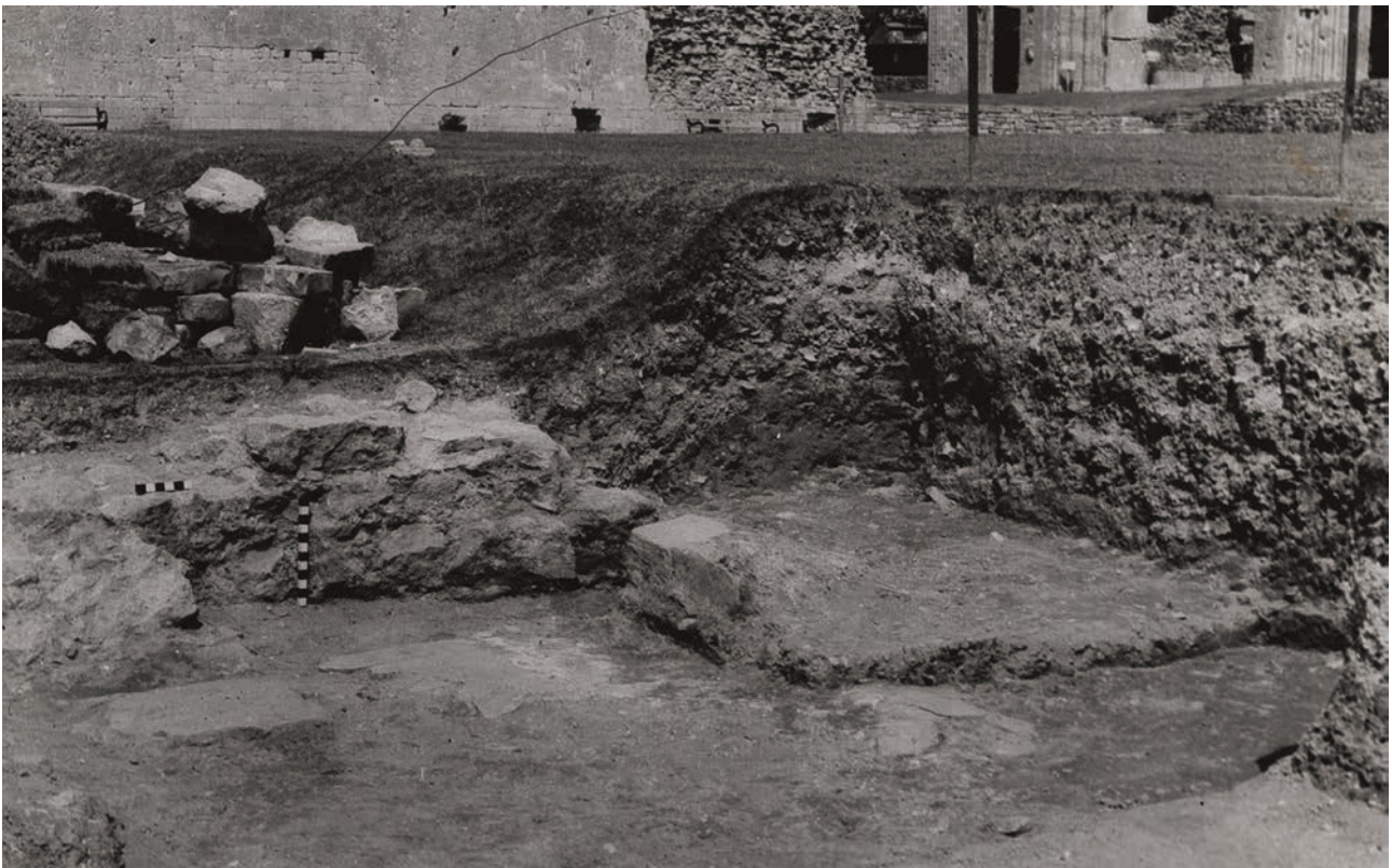
Fig 6.10 ?Wall of twelfth-century abbot's range, looking north east (1952 photograph: © EHA)
