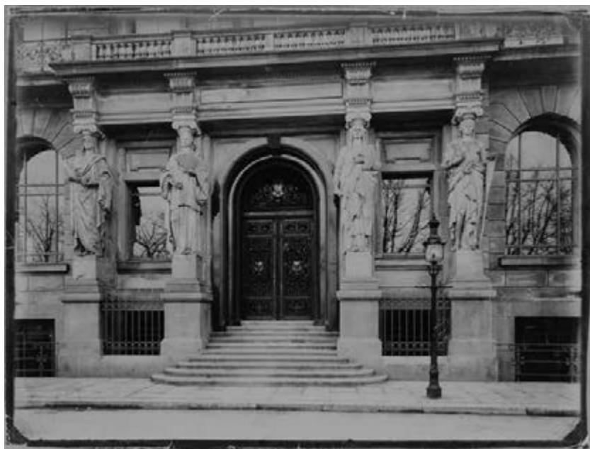
Figure 23 Photograph of the main entrance with the caryatids, representing from left to right Africa, Asia, America, and Australia. Encapsulated in the façade, they reminded clients and passers-by of the faraway worlds to which the office was connected in a globalised system of shipping and trade. The barefoot, bare-breasted statues of Africa and Australia contrasted with those of Asia and America, wearing shoes and clothes, following the conventions of portraying perceived differences in the level of civilisation.
