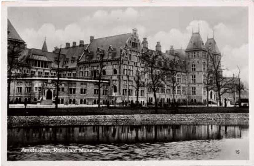
Figure 27 Amsterdam's Koloniaal Instituut seen from the north. The main entrance to the right gave access to an opulent marble rotunda, behind which the auditorium was located. The central part of the building visible here was home to offices, classrooms, laboratories, and storerooms, while a small part of the museum wing is just visible to the left. Note the references to Dutch Renaissance architecture, for instance in the shape of the gable.
