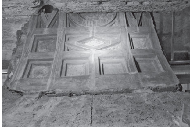
Fig. 10: Reconstructed ceiling block from room (3).
