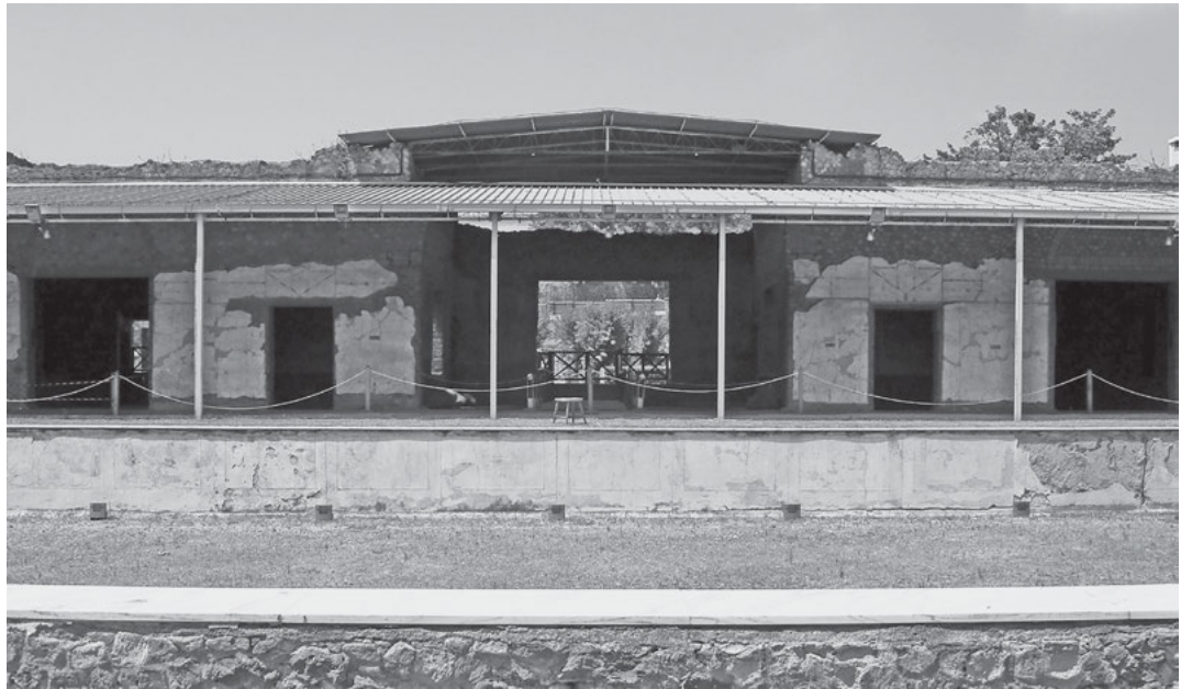
Fig. 10: Villa A at Oplontis, view of porticus (60) from the east side of the pool.
