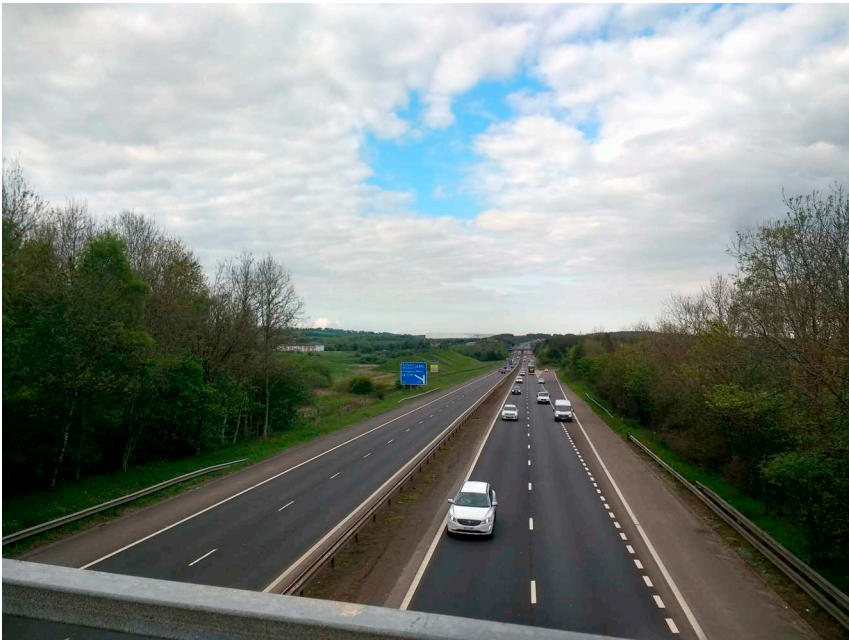
FIGURE 2.4 The M8 motorway, looking down the eastbound carriageway near junction 3a, back towards the outskirts of Livingston. Both the motorway and the town were built on thousands of tons of shale blaes extracted from nearby bings. Photograph by Jonathan Gardner, CC BY-NC 4.0.
