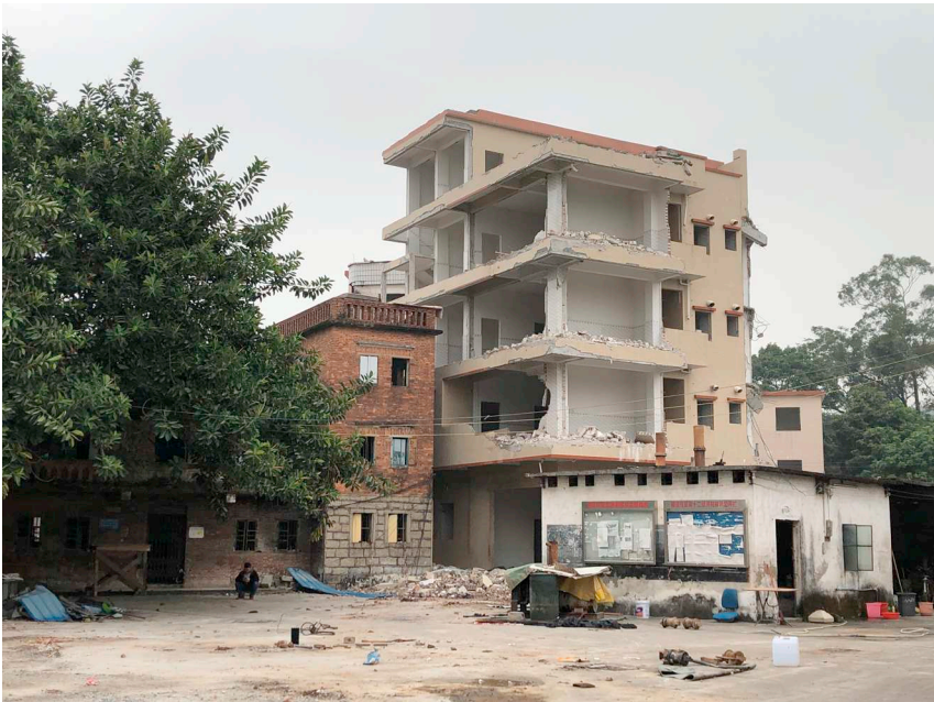
FIGURE 10.3 A standard three-level village house undergoing demolition.
