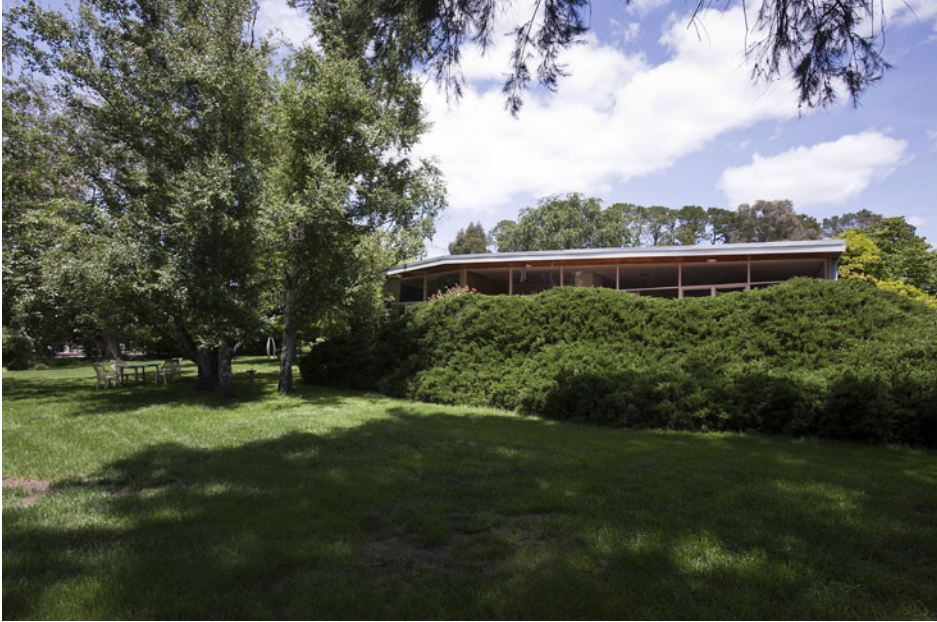
Figure 2.6 Fenner House, view from north-west
