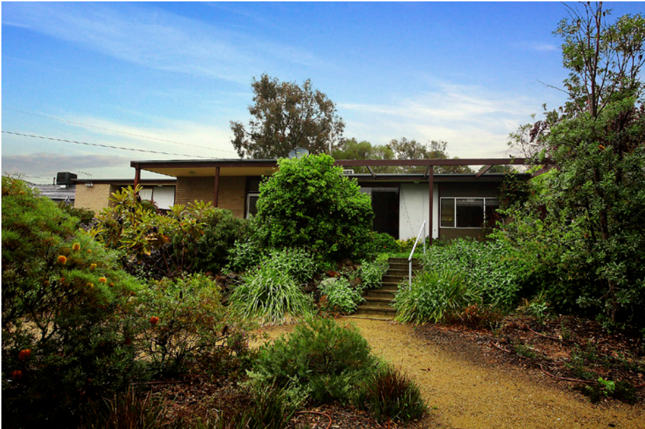
Figure 5.1 Gascoigne House, view from north
