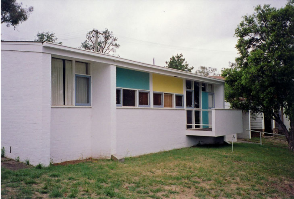
Figure 3.7 Zwar House, view from south
