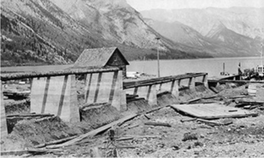
BUILDING THE NEW DOCK AT LAKE MINNEWANKA, 1912 (GLENBOW ARCHIVES, PD-365-2-10).
