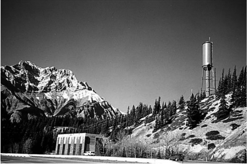
CASCADE POWER PLANT (AUTHOR PHOTO).
