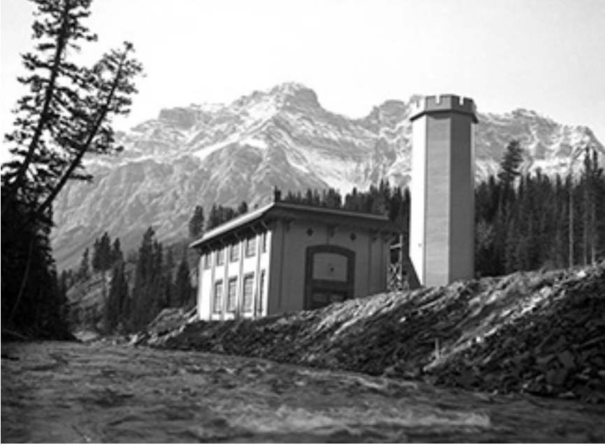
POWER STATION BUILT BY THE PARKS BRANCH AT LAKE MINNEWANKA (GLENBOW ARCHIVES, NA-841-396).
