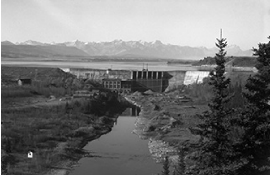
GHOST RIVER DAM NEARING COMPLETION (GLENBOW ARCHIVES, NA-4477-12).
