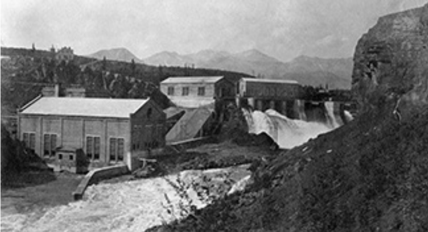
HORSESHOE FALLS POWER STATION (GLENBOW ARCHIVES, PD-365-1-93).
