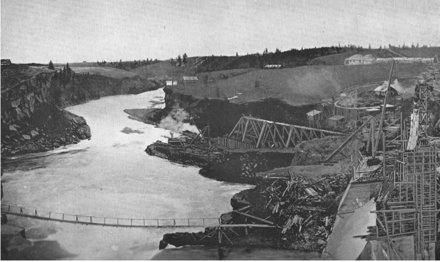
HORSESHOE FALLS POWER PLANT UNDER CONSTRUCTION, 1911 (COMMISSION OF CONSERVATION).
