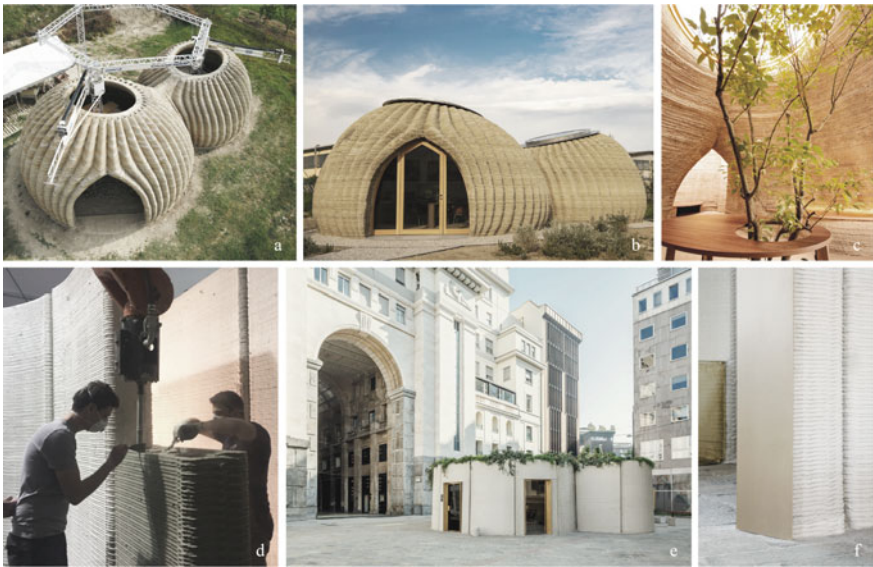
Fig. 28.2 ‘Here and Now,’ instant architecture. TECLA—Technology and Clay is a project by MCA—Mario Cucinella Architects and WASP (a ©WASP, b, c ©Iago Corazza). 3DHousing05 is a project by Locatelli Partners (d–f ©Luca Rotondo, courtesy Locatelli Partners)
