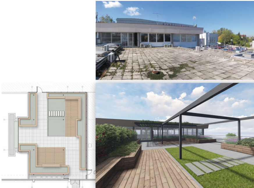
Fig. 75.3 Zone 2—roof terrace above the entrance hall—existing state (top), top view (bottom left), and rendering (bottom right)
