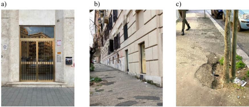
Fig. 85.2 Walkways in the case study. a An architectural barrier at building entrance in Via Urbino. b Irregular surfaces in Via Fregene. c Incompliant gaps in Via Veio
