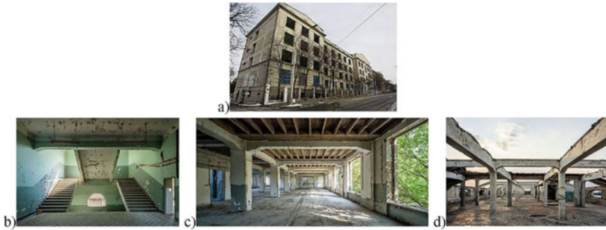
Fig. 73.1 “Beko” building before reconstruction: a street view (Author Đorđe Kojadinović, RAS Srbija), b–d interior and structure. (Source Remorker Architects)
