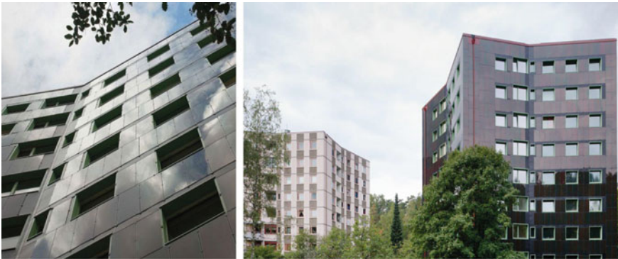
Fig. 29.13 Renovation of Stacken apartment building
