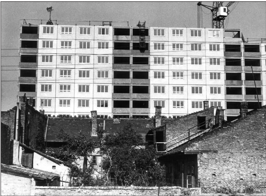
Figure 21. The building of prefabricated panel houses in Óbuda, Budapest in 1970. From the early sixties, the construction of housing estates, based on prefabricated block technology, helped to alleviate the housing shortage (Fortepan, 47344, Óbudai Múzeum)
