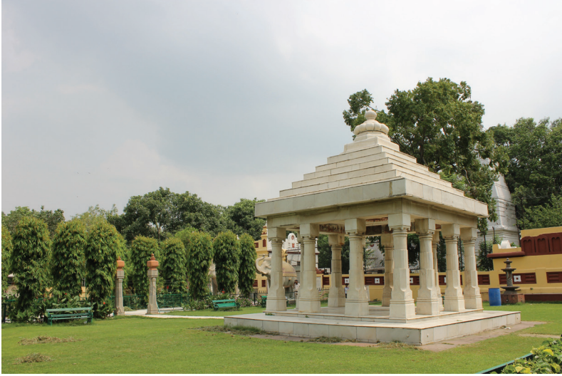
Figure 6.3 The wedding maṇḍapa in the grounds of the Lakshmi Narayan temple, New Delhi. © Agnieszka Staszczuk.
