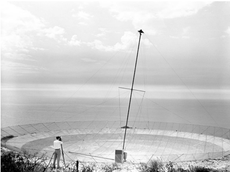
Fig. 23.5 Another striking photo of the 80-foot aerial, possibly with either Dick McGee or Gordon Stanley measuring the position of the feed, view to the east over the Tasman Sea. Credit: CSIRO Radio Astronomy Image Archive B3150-2
