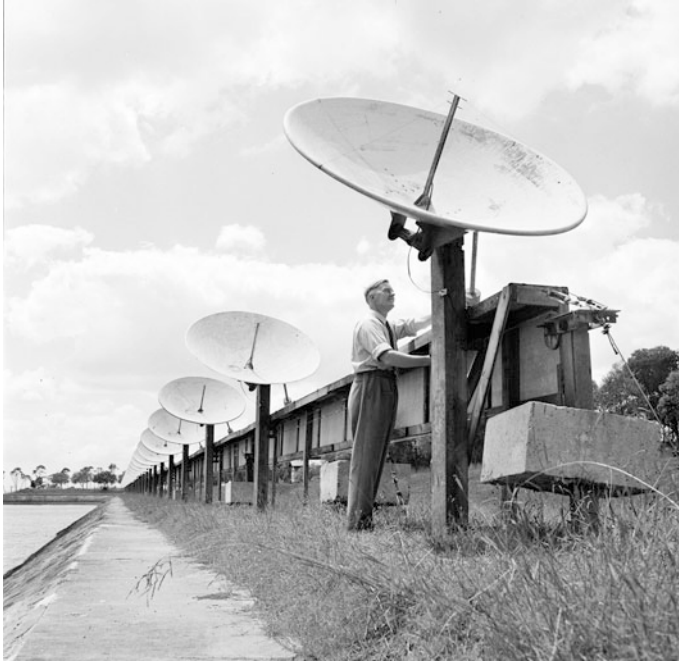
Fig. 37.9 (Chris) Christiansen and his 32-element solar array at Potts Hill Reservoir 1953. Credit: CSIRO Radio Astronomy Image Archive 2976-1
