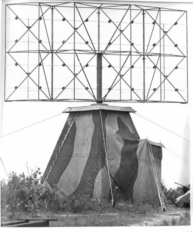
Fig. 9.3 The initial aerial (LW/AW) in late 1942. The aerial was a 32-element array of half-wave end-fed dipoles. The feeder system used 330 ohm twin transmission lines (developed by Pawsey). The modest canvas tent contained the transmitter and receiver, with cramped quarters for the operators. The tent was made at Chullora Railways Workshops, near Lidcombe, a Sydney suburb. Credit: CSIRO Radio Astronomy Image Archive JP09–3
