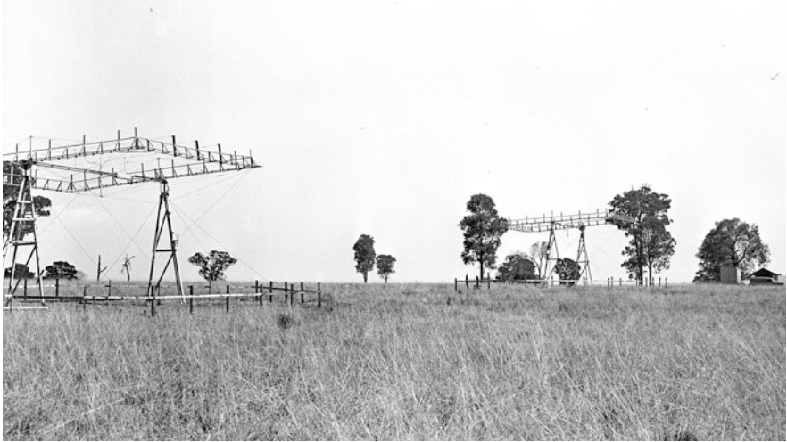
Fig. 21.1 Two of the three elements used for the 101 MHz all sky survey made by Mills in 1950–1951. The three elements were spaced by 60 m and 270 m, giving lobe spacings of 3^\circ and 40 arc min. This is the 60 m spacing. With two spacings a rough estimate of the angular size of the radio sources could be detected. The same antennas were used for the sky survey as discussed in more detail in Chap. 33. Credit: CSIRO Radio Astronomy Image Archive B2594-3
