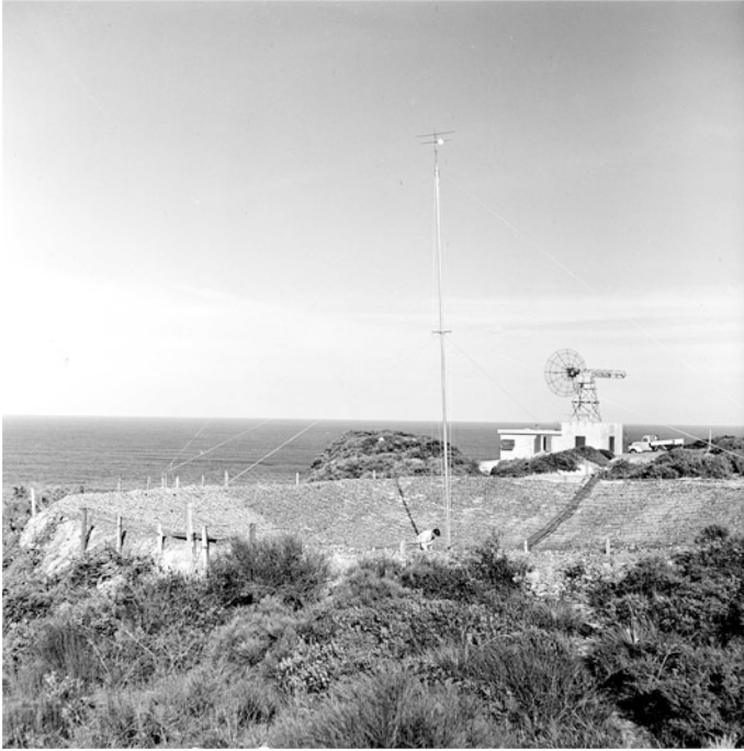
Fig. 23.2 In the foreground is the 72-foot hole-in-the-ground built in 1951 for a survey of the region near the galactic centre at 160 MHz. In the background is the 16-foot reflector built in 1950 mainly for instrument development in the decimetre wavelength range. Credit: CSIRO Radio Astronomy Image Archive B2763-1
