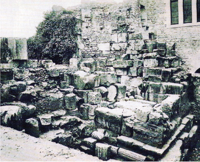
Figure 4.10: Foundation of tower C, late antique city wall of Périgueux. Photograph: Ch. Durand, 1920.
