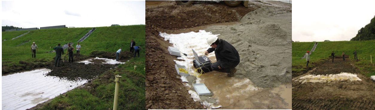
Figure 3. Installation of a non-woven geotextile containing single-mode silica fibers as Brillouin sensors in a gravity dam in Solina, Poland.
