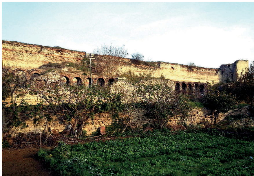
Fig. 5: Casemates of the Outer Wall, Photo: N. Asutay-Effenberger.
