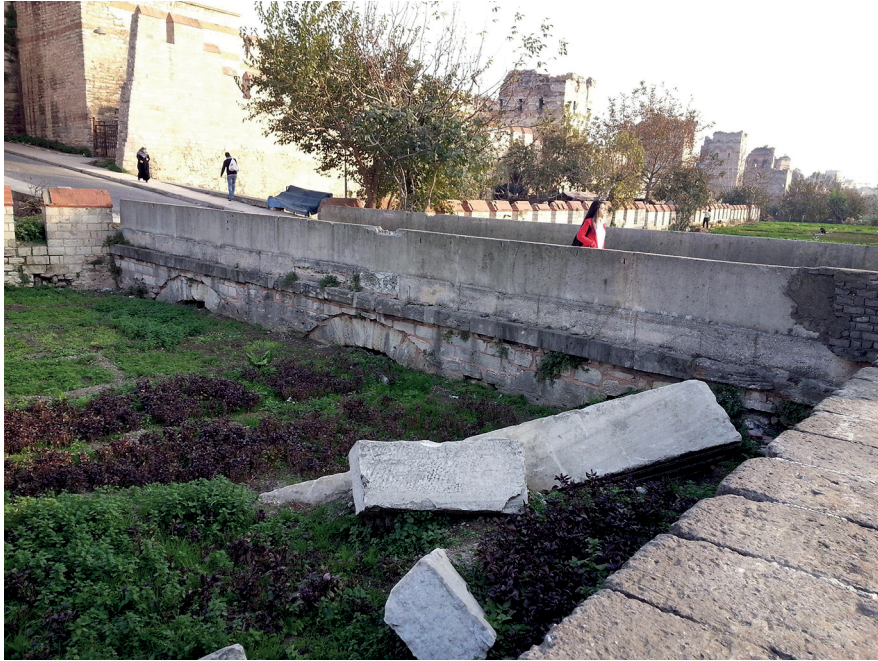
Fig. 7: Bridge at the Belgradkapı, Photo: N. Asutay-Effenberger.
