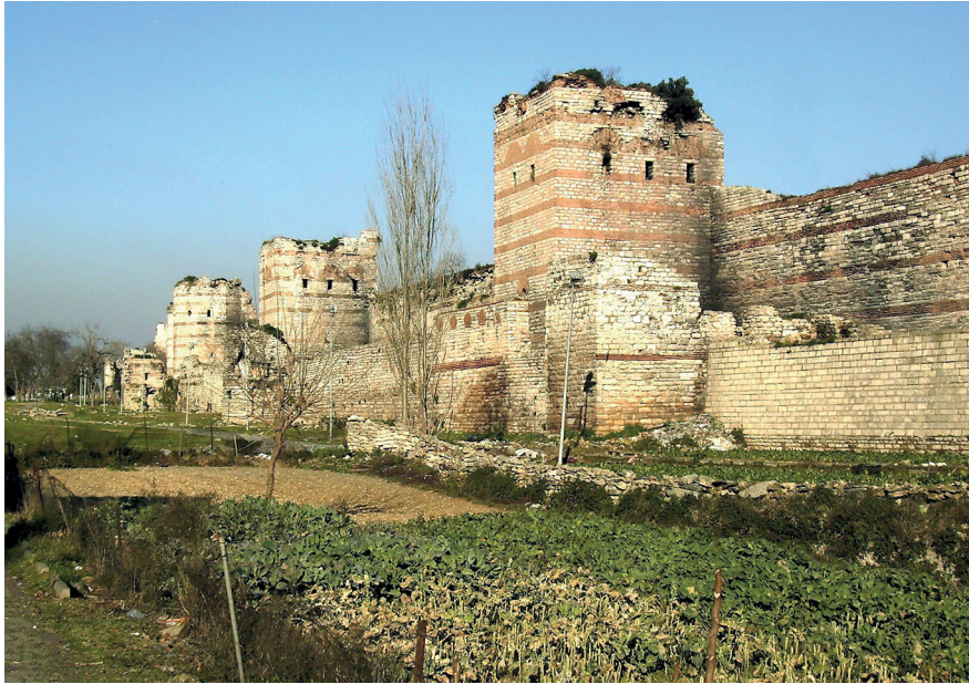
Fig. 2: Theodosian Land Walls, Main Wall, Outer Wall, Outer Ward and the Moat, Photo: N. Asutay-Effenberger.
