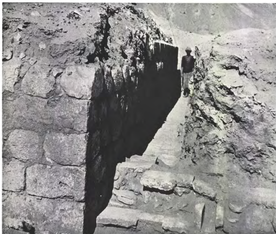
East corner of platform, phase 'A', looking north. Workman stands on phase 'C' pavement
