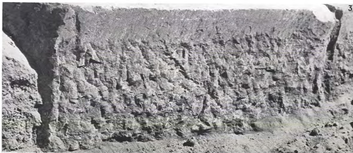
Detail of stone dressing on coping of phase 'B'
