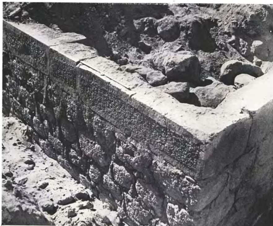
Coping at north corner of phase 'A' platform, with boulder fill
