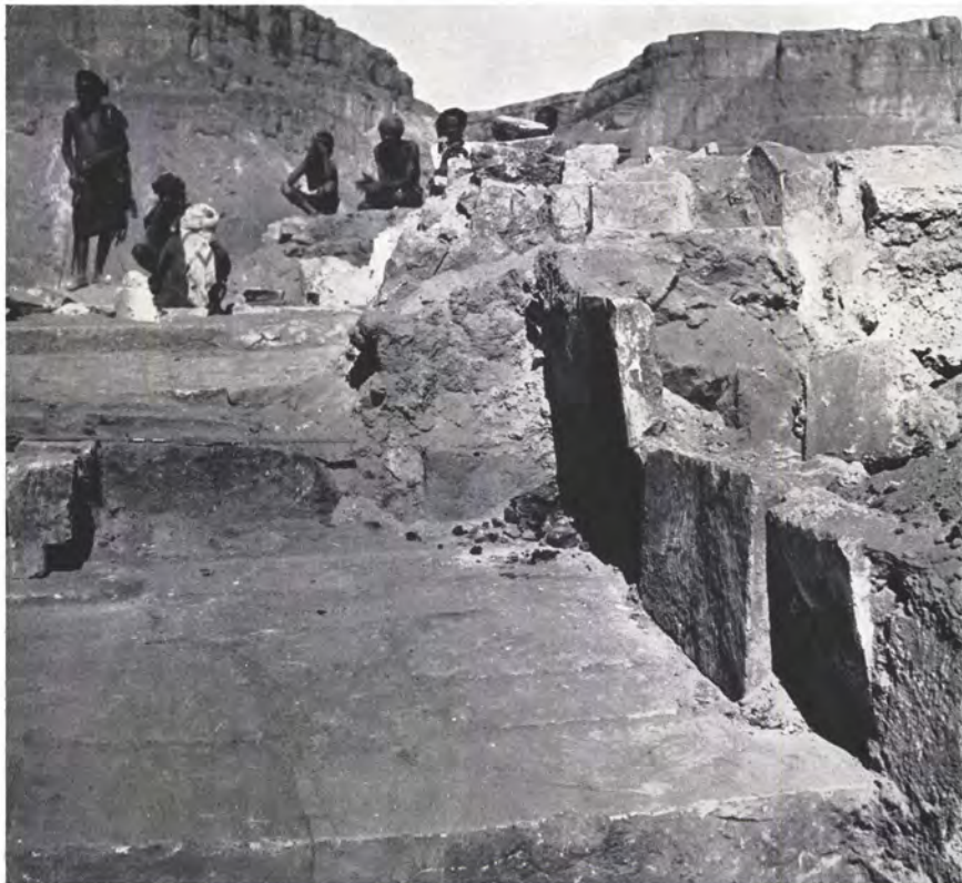
Forecourt area VIII at head of south-east steps with stone dado and (left) drain. All phase 'C'. Bedouin spectators to rear
