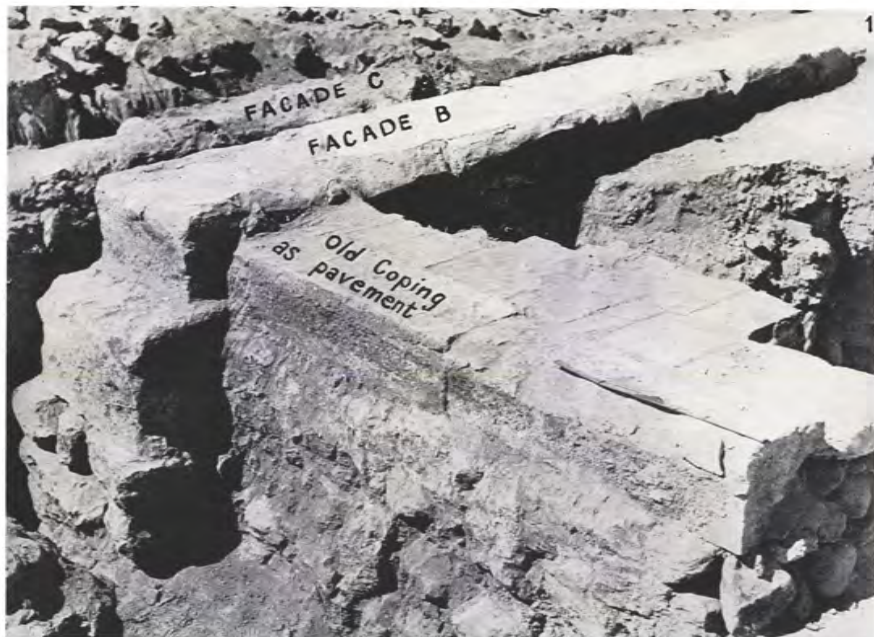
The two 'false' façades of phases 'B' and 'C'. Foreground: shallow cross-wall with old copings re-used as pavings
