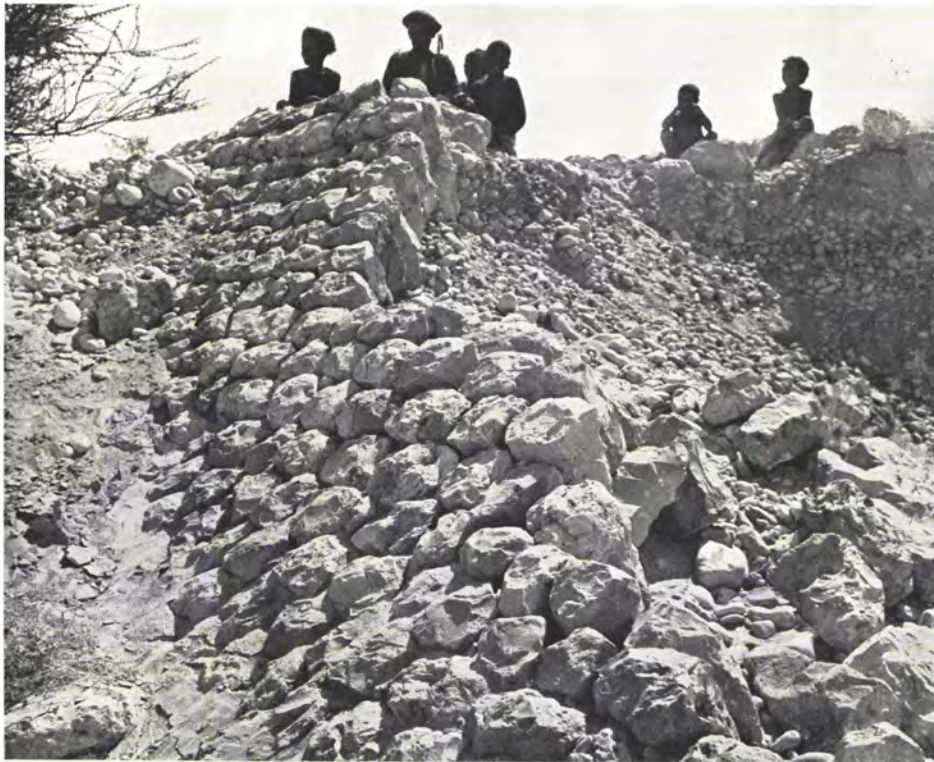
Revetment of dam
