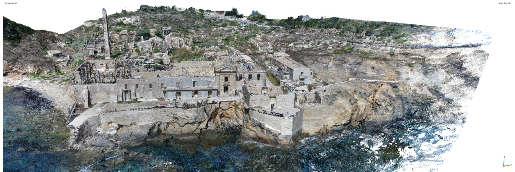
Fig. 5. Point cloud models of the buildings of the Capo Passero tonnara.
