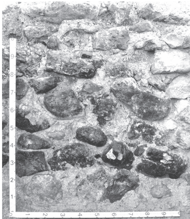
Fig. 252 Soot on northern wall of Room 19
